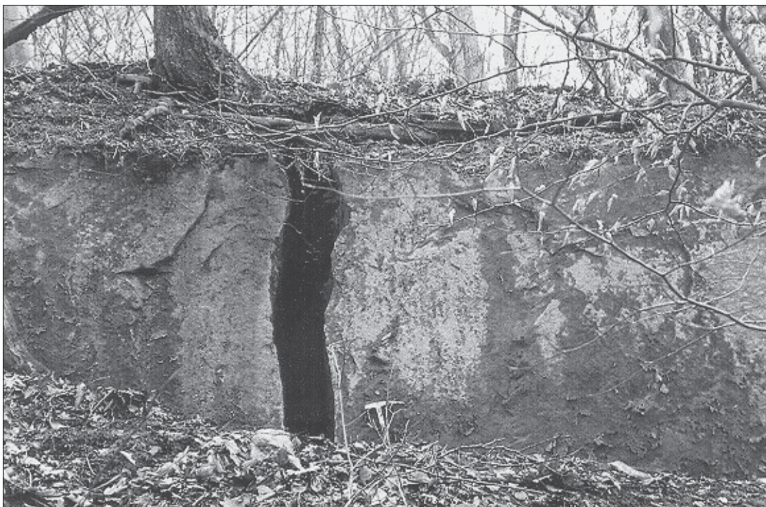
FIGURE 16.—Vertical subsidence fracture in the Lower Freeport sandstone overlying the Majestic Mine. Rock hammer at bottom center for scale.
