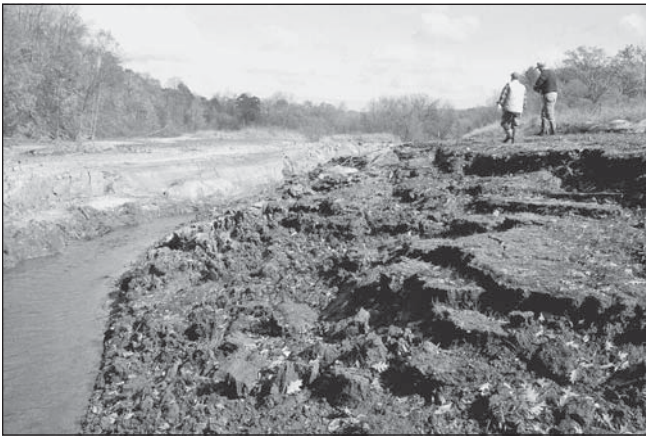
FIGURE 8-5.—Channel incision and slumping of reservoir sediments immediately following the dam failure, as the Chagrin River restores its channel shape and slope to the breaching of the dam. Photo by J. Evans.
