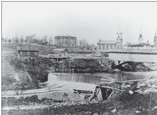
FIGURE 9-11.—Dam and associated (lower) lock along the Cuyahoga River, Kent, Ohio, circa 1870. The canal prism (ditch) is in the foreground, on the east side of the Cuyahoga River, and the lock is to the bottom right. The old (1837) stone-and-wood covered bridge over the Cuyahoga is seen in the middle right. The current Main Street Bridge replaced that bridge in 1877. Photograph courtesy of Archival Services, University of Akron.
