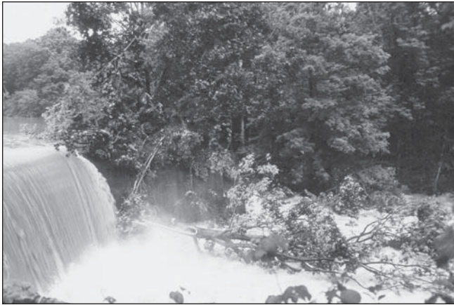
FIGURE 8-2.—Photograph of the spillway of the IVEX Dam minutes before failure of the dam at the spillway–earth-fill dam contact (right). Photo courtesy of Y. Rausch, Chagrin Falls Historical Society.
