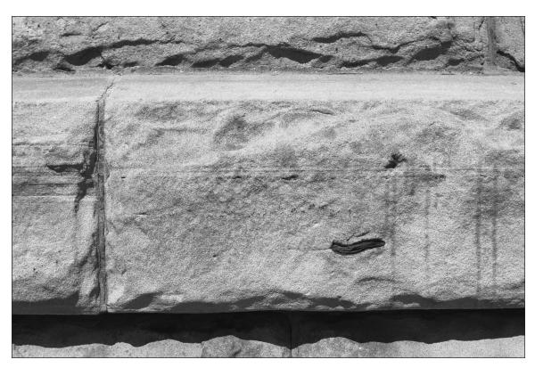
FIGURE 53.—Detail of stone used for the exterior of St. Bernard's Church. A large clayey clast can be seen in the large block. April 2005 photo.
