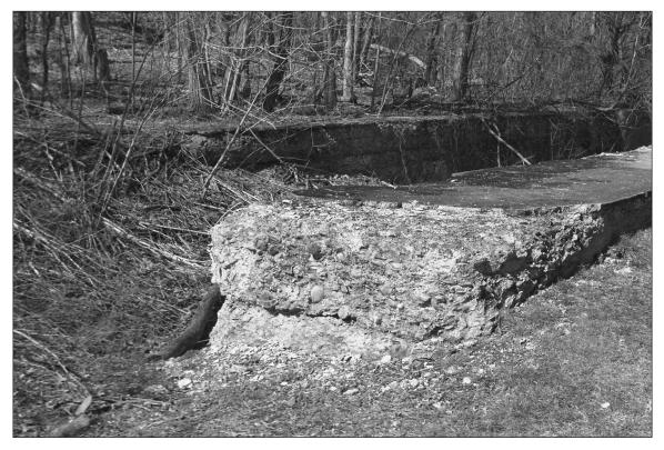
FIGURE 45.—Upper end of Lock 16, north of Mustill Store. Note weathered surface, exposing rounded and other stones used in the concrete walls. April 2005 photo.
