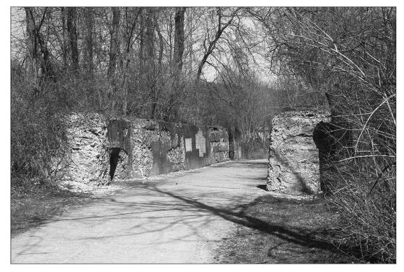
FIGURE 47.—Upper end of Lock 18, Akron, north of Mustill Store. The towpath trail passes through this concrete lock, allowing the concrete of the inner lock walls to be easily examined. April 2005 photo.
