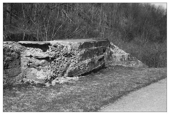
FIGURE 46.—Lower end of Lock 17, north of Mustill Store. Note large slab of protruding sandstone (arrow) included in the concrete used for the lock, as well as the indications of the forms used to contain the concrete when first poured. April 2005 photo
