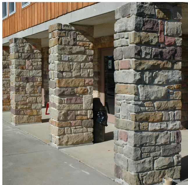
FIGURE 22. —Columns of multicolored sandstone at the Shawnee State Park Marina in Scioto County, Ohio, are typical of the Pennsylvanian Massillon sandstone quarried by Briar Hill Stone Company in Coshocton County, Ohio.
