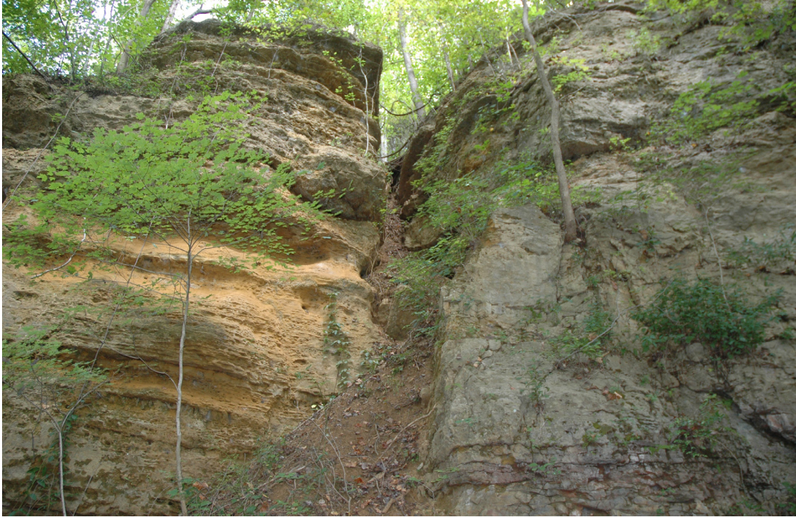
FIGURE 34.—Approximately 50 ft of the Peebles Dolomite and Lilley Formation are exposed north of U.S. Rte. 52 in Adams County, Ohio. Note the solution-enlarged, near-vertical joint.
