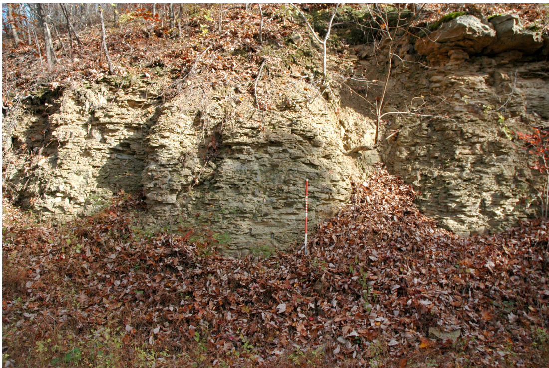
FIGURE 25.—Road cut on Shawnee State Forest Rd. 5, Scioto County, Ohio. Exposed is the top of the Byer Member of the Logan Formation. Note the repetitive, medium- to thick-bedded, sparsely fossiliferous siltstone beds that indicate a marine shelf depositional environment. The surveying rod is 5 ft high.
