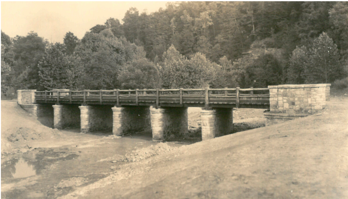
FIGURE 5.—An example of the superb stonework completed by the Civilian Conservation Corps (CCC) in the Shawnee State Forest, Ohio, circa 1938. This bridge crossed Turkey Creek just below Roosevelt Lake Dam. The piers and abutments were removed and replaced with a modern bridge in 2016. An original pier and an abutment were retained and used to create a memorial, placed at the shelter house on Mackletree Road, to the African American CCC workers who constructed the bridge (Charles Egbert, ODNR Division of Forestry, written comm., 2018). Photo courtesy of ODNR Division of Forestry.
