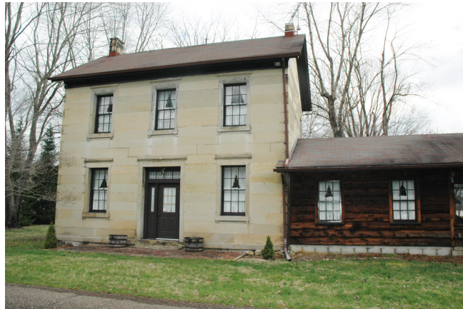
FIGURE 32. —Restored stone house (private residence) on the Ohio River at Buena Vista, Ohio. The building was constructed using local building stone and was the office of the Buena Vista Freestone Company during the 1800s.
