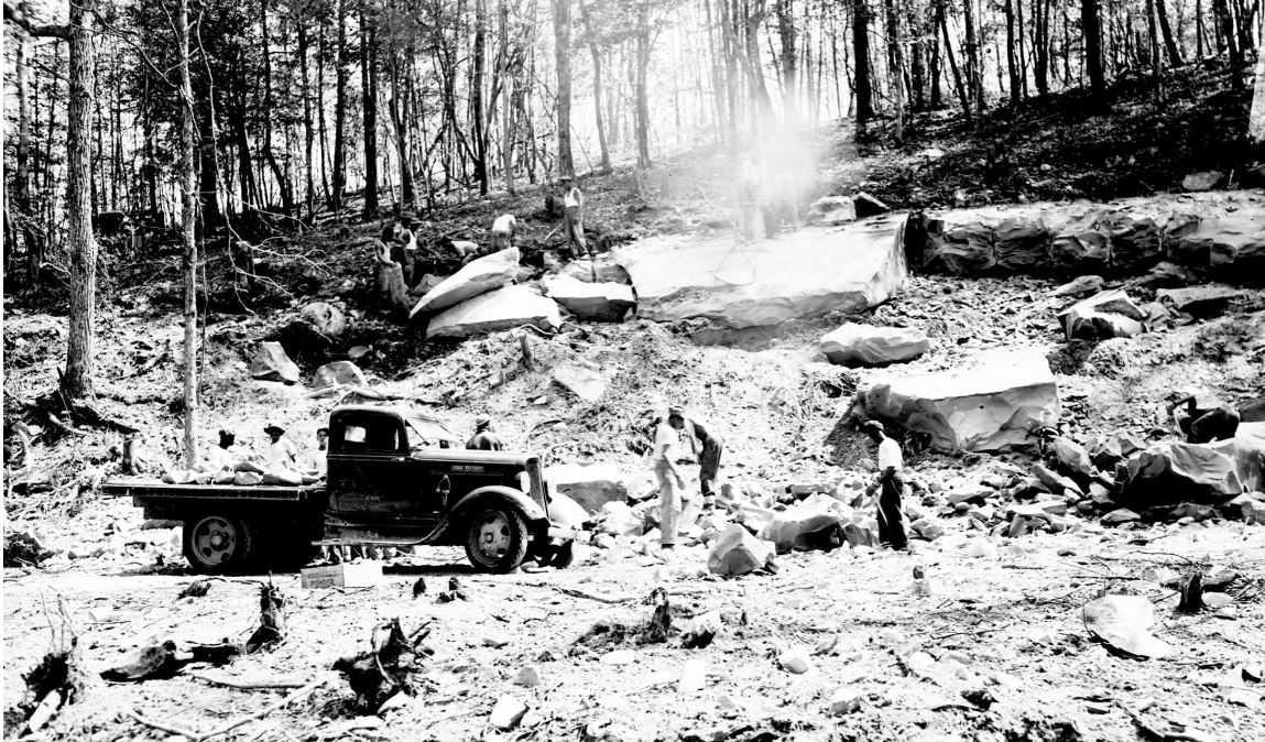
FIGURE 4.—Civilian Conservation Corps crew drilling and blasting large slabs of sandstone to be used for construction of roads, bridges, and other structures in Shawnee State Forest, Ohio, circa 1930s. Photo from the Ohio Agricultural Experiment Station, Department of Forestry collection at Ohio State University.
