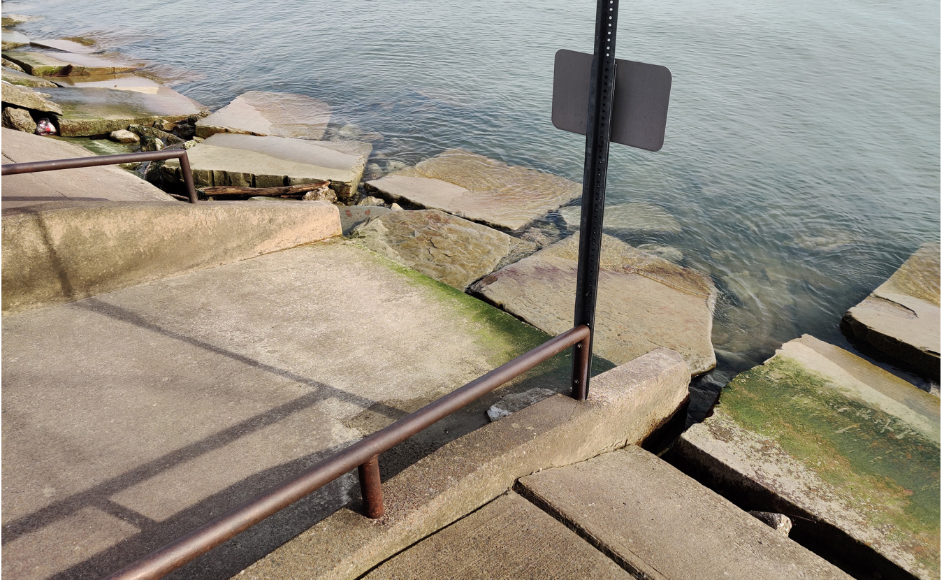
FIGURE 45. Ramp at East Harbor State Park, Ottawa County, Ohio, that once led to a sand beach (see fig. 44) but now leads only to water.
