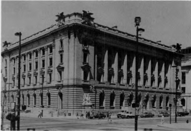
FIGURE 12.—Old Federal Building at Superior Avenue and Public Square, faced with very light gray Mount Waldo granite . Photo circa 1988.
