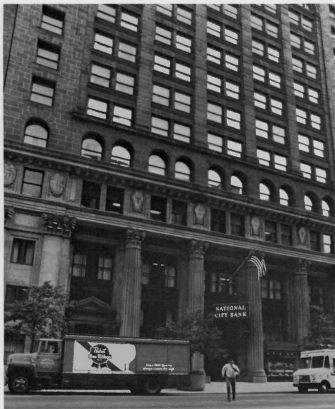
FIGURE 30.—National City Bank Building. The lower portion of the building is faced with Stony Creek Red granite .
