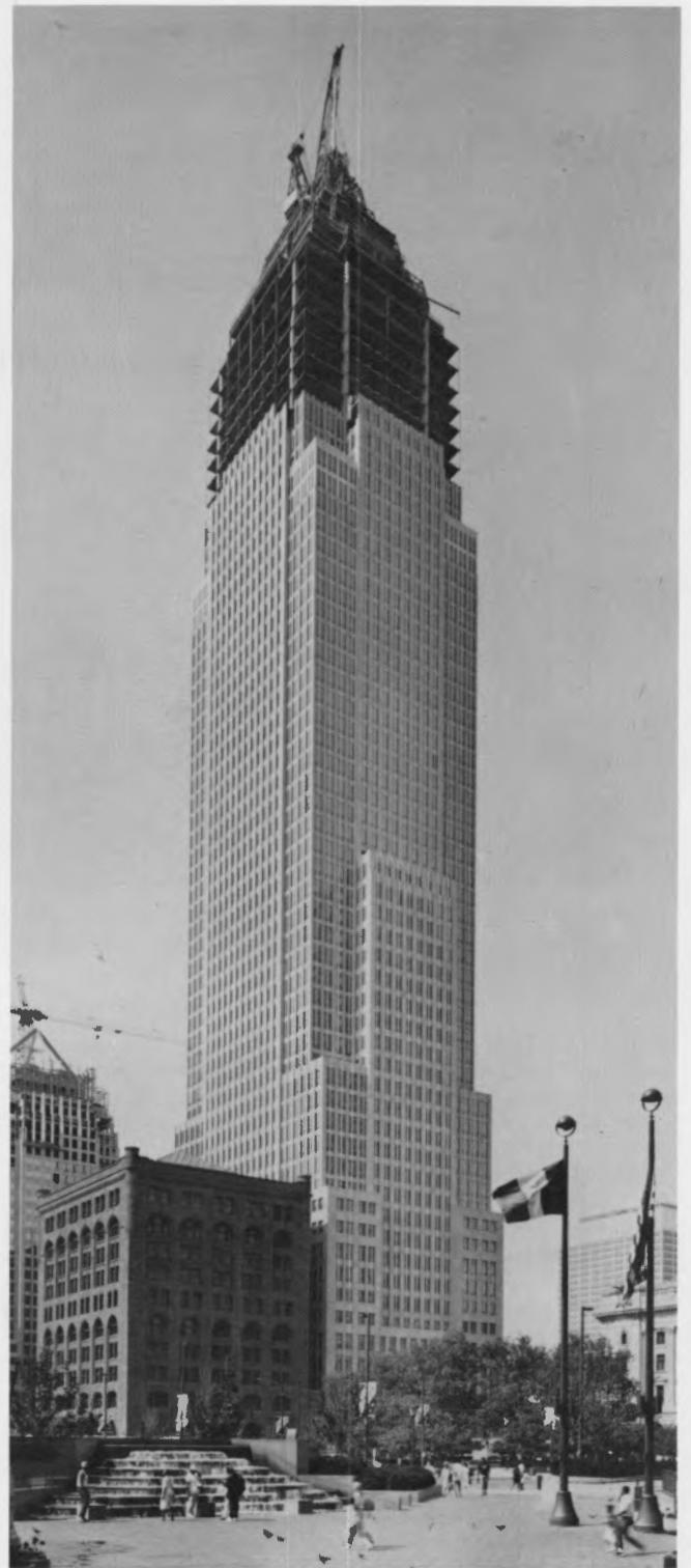
FIGURE 11.—Society Tower, as it was being completed in 1991. The stone facing visible in this photo is Stony Creek granite . The Society for Savings Building is to the left of the Society Tower. Because its exterior was recently cleaned, the color of the stone walls of the Society for Savings Building appears to be lighter than in figure 10. Photo by M. Vantz, The Cleveland Electric Illuminating Company, 1991.
