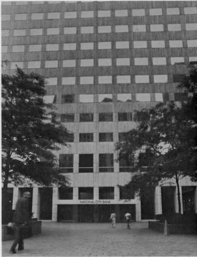
FIGURE 28.—National City Center Building. Facing of white travertine shows differential darkening, probably due to pollutants.
