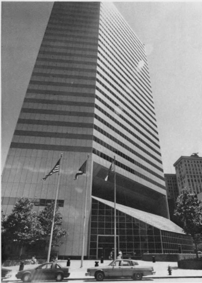
FIGURE 24.—One Cleveland Center. Dark-gray Crown Point Limestone is used around the base of the building.
