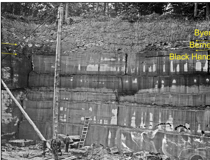
Figure 3. Historic photograph of Sharp Quarry, Sugar Grove, Ohio (J.E. Hyde, 1904–1905). The quarries at Chestnut Ridge would have looked similar to this at the height of production. The lowermost unit is the Black Hand Sandstone.
