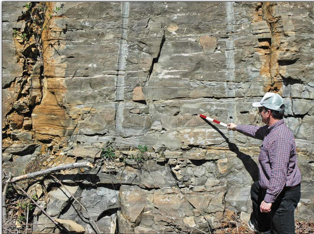
Cross-bedded and cross-laminated, fine-crystalline, fossiliferous dolomite of the Bisher Formation exposed in a road cut for S.R. 41 south of Peebles, Adams County. This cut contains prominent oxidized, solution-enlarged, vertical cracks. Scale is 50 cm (1.6 ft) and is pointing to shale rip-up clasts.
