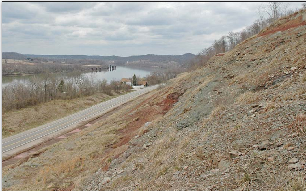
Dunkard Group red beds, gray shale and clay beds, and thin sandstone beds in road cut for S.R. 68 just north of Sherman, West Virginia, and east of Buffington Island, Meigs County, Ohio.
