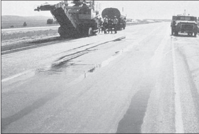
Rutting of an asphalt pavement and resulting ponding. From Distress Identification Manual for the Long-Term Pavement Performance Project, Strategic Highway Research Program, National Research Council, National Academy of Sciences, 1993. Used with permission.
