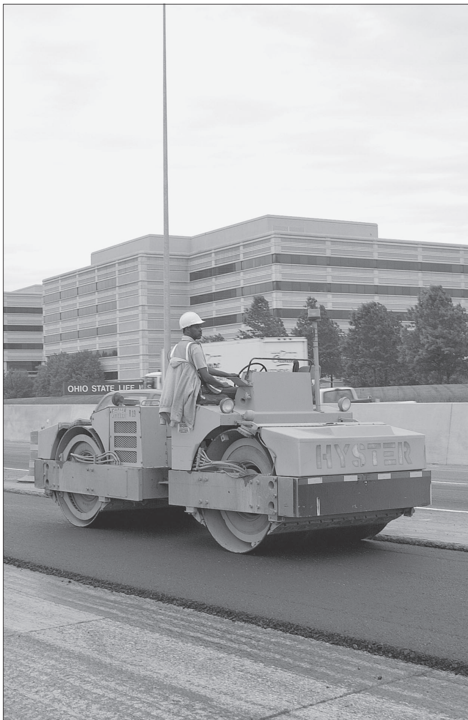
Roller operator Jerome Slaughter of The Shelly Company smoothing and compacting recently installed asphalt pavement. The location is immediately east of the I-270 and Sawmill Road interchange in northern Franklin County.
