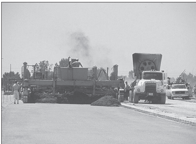
Portland concrete paving in progress. The concrete is transported from the mixing plant by truck. Photo courtesy of the Ohio Ready-Mixed Concrete Association.
