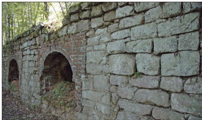
Close-up of the Cherry Valley coke ovens near Leetonia, Columbiana County, Ohio, illustrating the use of locally-sourced sandstone for foundations and bricks produced from area clays and shales used to construct and line the ovens. Coal mined nearby was the raw material for the coke ovens and native iron-ore was used in the furnaces.
