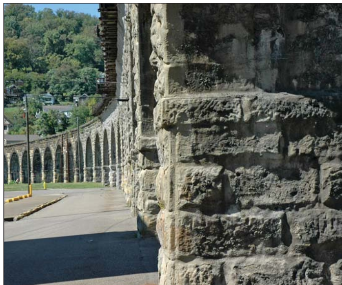
West-facing view of the B. & O. Railroad viaduct at Bellaire, Belmont County, Ohio. The viaduct was constructed in 1870 using Pennsylvanian-age “Bellaire sandstone” quarried to the north at Martins Ferry, Ohio (Camp, 2006). The Bellaire viaduct consists of 43 arched spans leading to the railroad bridge crossing the Ohio River; the bridge is supported by an additional six sandstone piers and abutments. More than 50,000 tons of stone was used during construction. Prior to building the bridge and viaduct, rail cars had to be ferried across the Ohio River.
