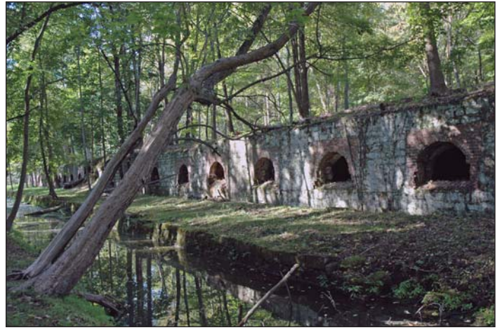
Some of the remaining 120 coke ovens of the original 200 constructed by the Leetonia Iron & Coal Company from 1866 through 1870 in Columbiana County, Ohio. The Cherry Valley Iron & Coal Company began operating the coke ovens and nearby iron furnaces in 1872.
