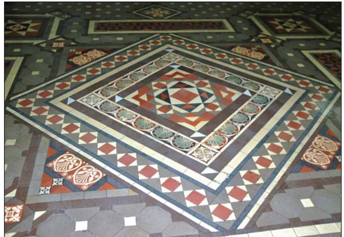
FIGURE 1. View of the ceramic tile floor in the rotunda of the Muskingum County Courthouse in Zanesville, Ohio. The courthouse floor was installed in 1877 by the Zanesville-based company, Fisher and Lansing, and is the oldest surviving American-made ceramic tile floor in the United States. The photo was taken in 2014; the tile floor displays remarkable longevity for a public building with 137 years of continual foot traffic.
