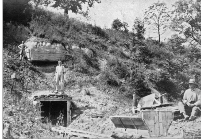
FIGURE 4. Carl Crabtree mine located on Blunt Run north of Zanesville in Muskingum County, Ohio. The Pennsylvanian-age Tionesta clay was being mined. Notice the outcropping Putnam Hill limestone approximately 15 feet above the mine entrance. Photo circa 1920.
