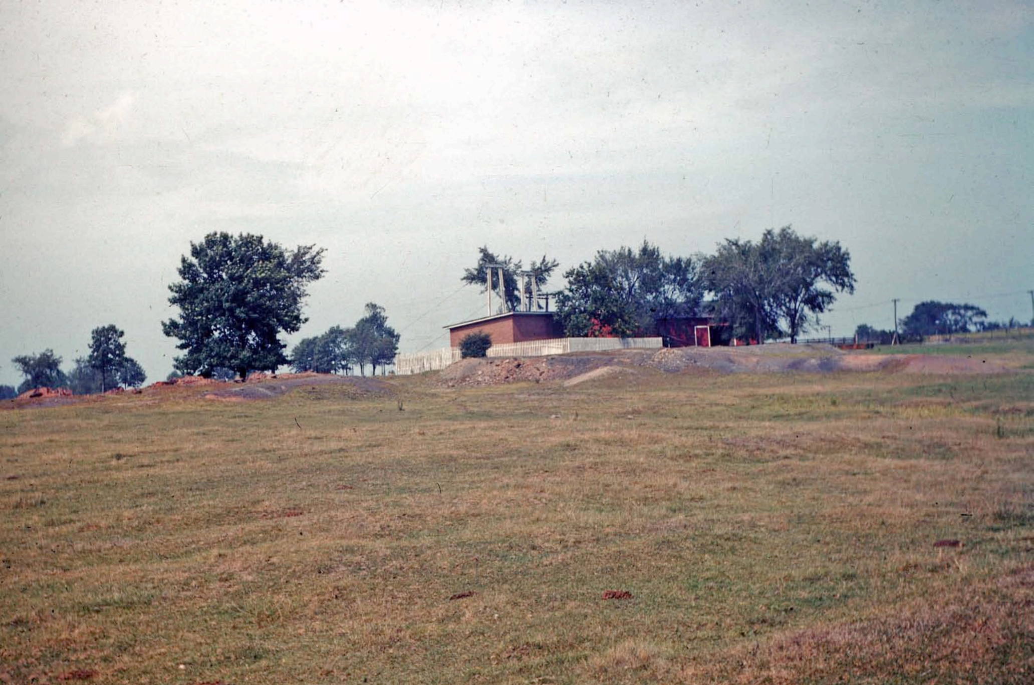
Weathersfield Pumping Station, Mineral Ridge, Ohio.
