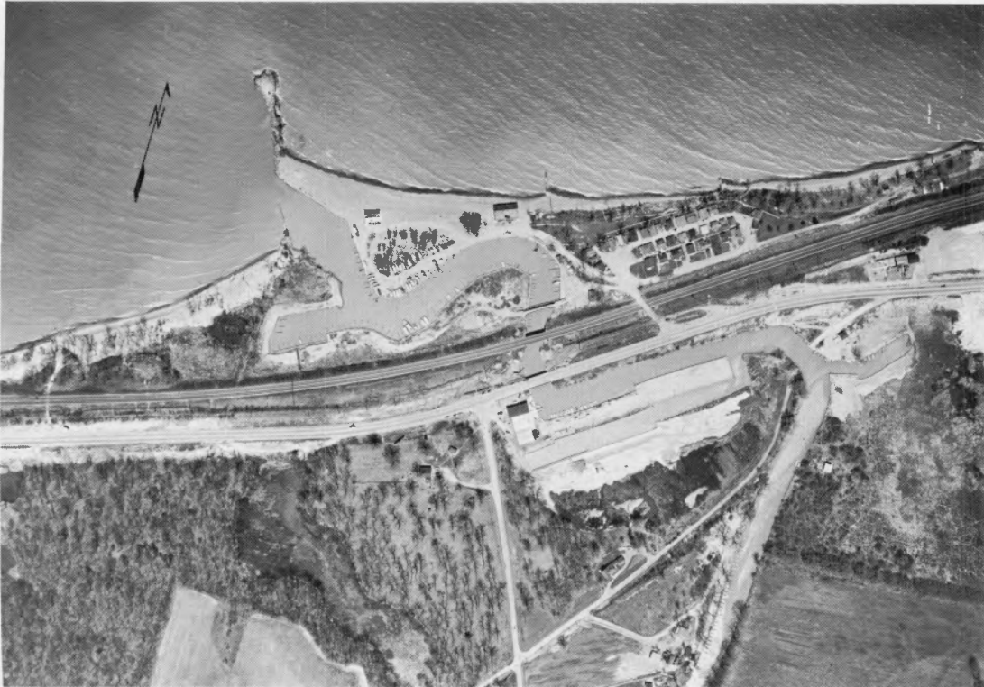
Figure 11.- Beaver Creek, four miles east of Vermilion, Ohio. Beaches east and west of creek mouth jetty are relatively stable. Jetty retains beach to east. Photo taken 5/7/56. Water level 573.2.
