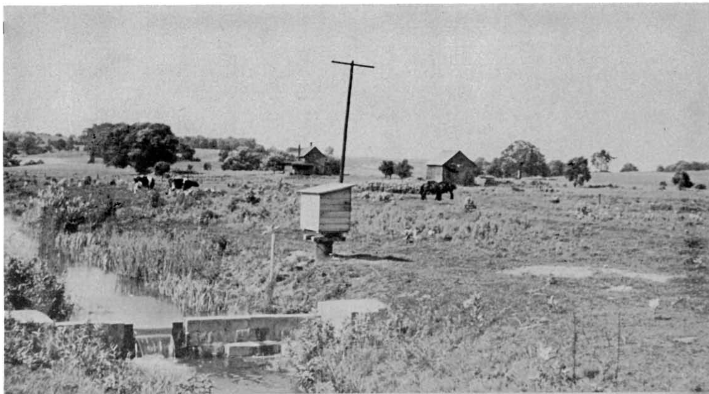
WEIR WITH RECORDING GAGE IN SHELTER TO RECORD FLOW OF SIPPO CREEK DURING PUMPING TEST.
