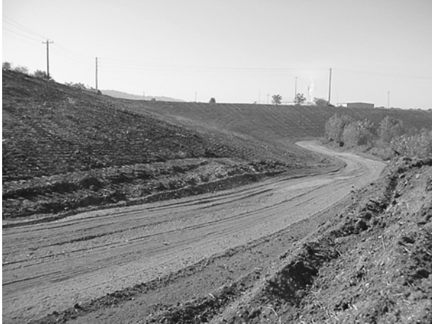
Land disturbed by mining activities is graded in preparation for seeding.
