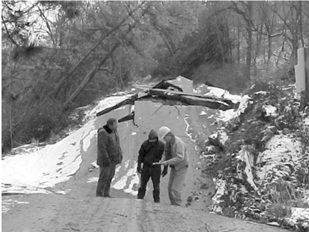
A landslide caused by a coal mining operation required immediate enforcement measures.
