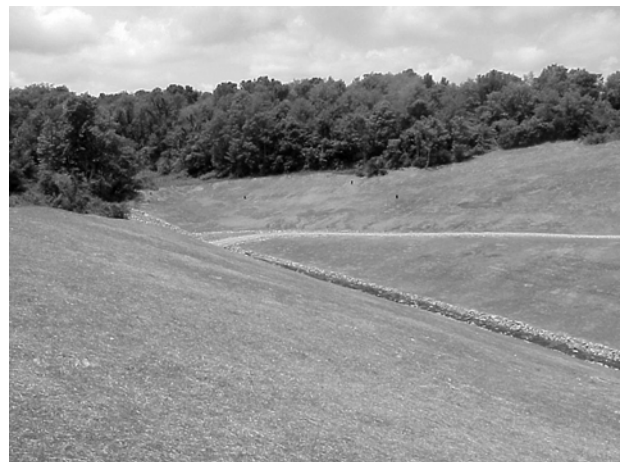
A reclaimed forfeiture site in Belmont County is restored to a productive condition.
