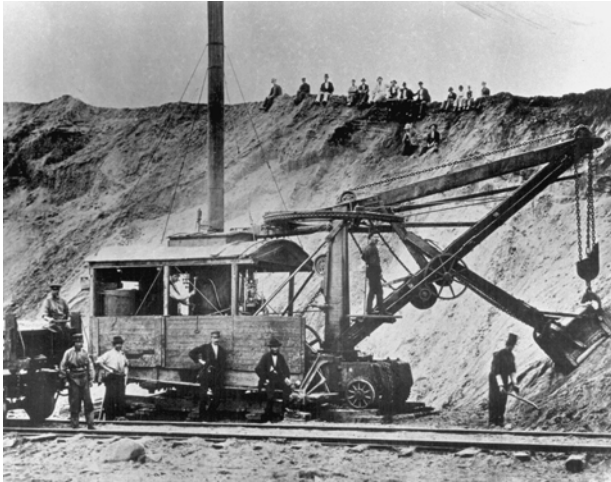
A coal-fired steam shovel that operated on rails. Circa 1890s.
