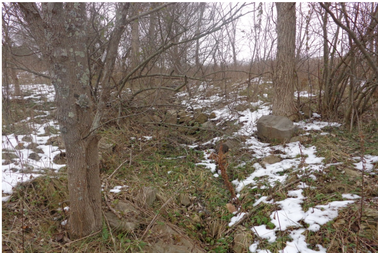
C-0209 (12-1-2013) – midstream looking upstream of reconstructed channel
