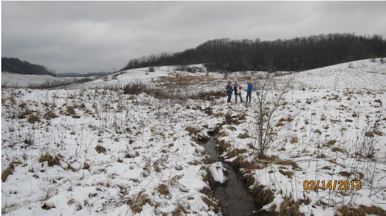
D-0807– planning work for reconstructed stream channel
