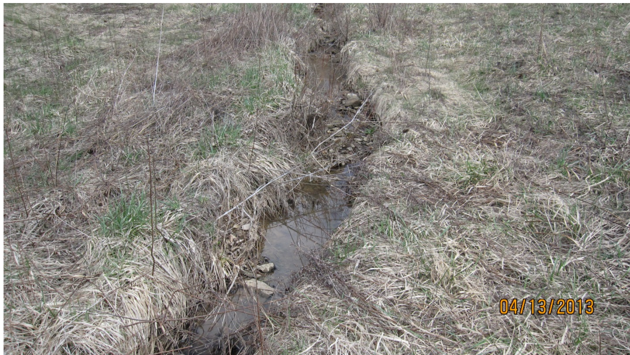
D-0807– view of reconstructed stream substrate
