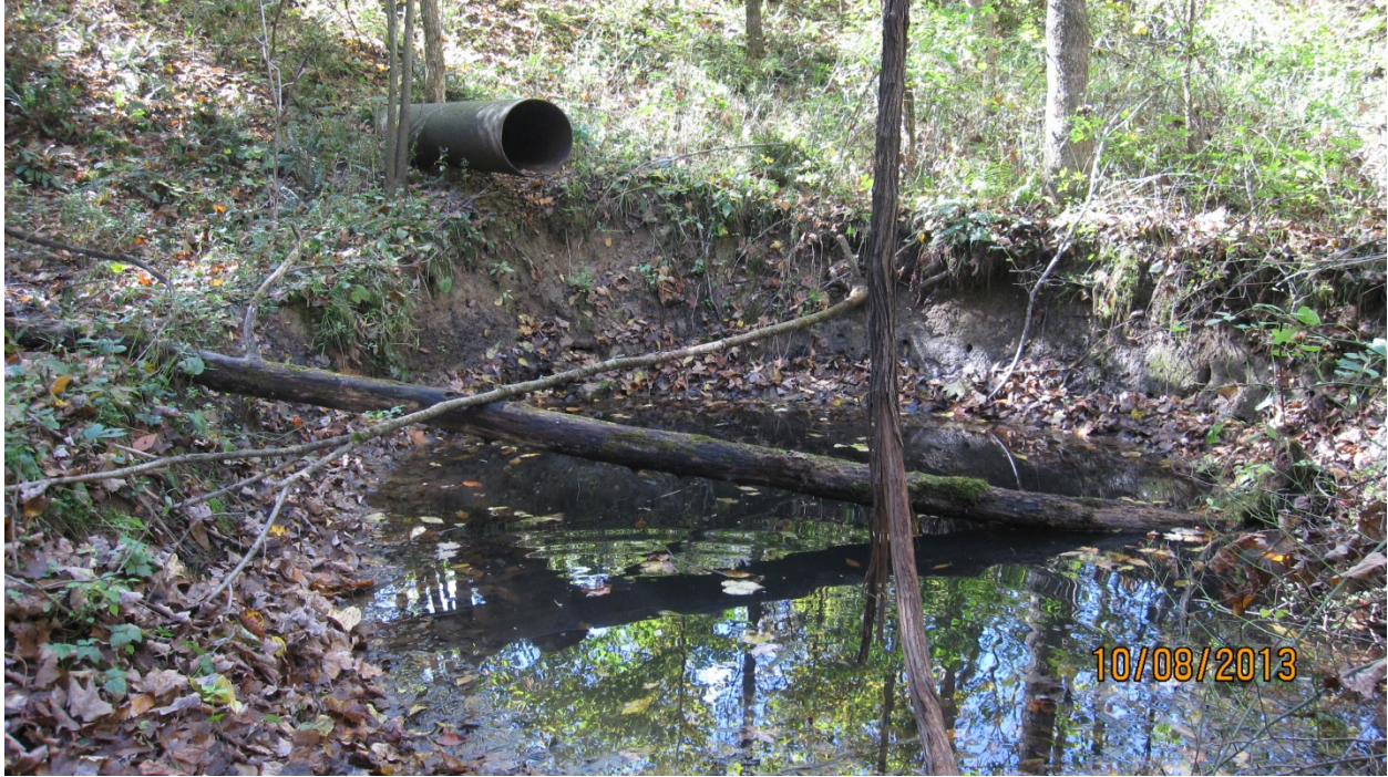
D-019 Bio- pond outlet and plunge pool at the head of the biological segment
