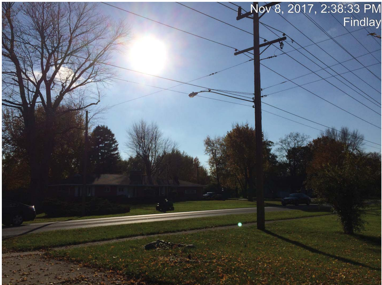
Photo of the Rice #1 looking to the south. Note that the well is located directly under the overhead electric lines.
