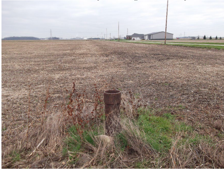
Randy Boes #1 wellhead
