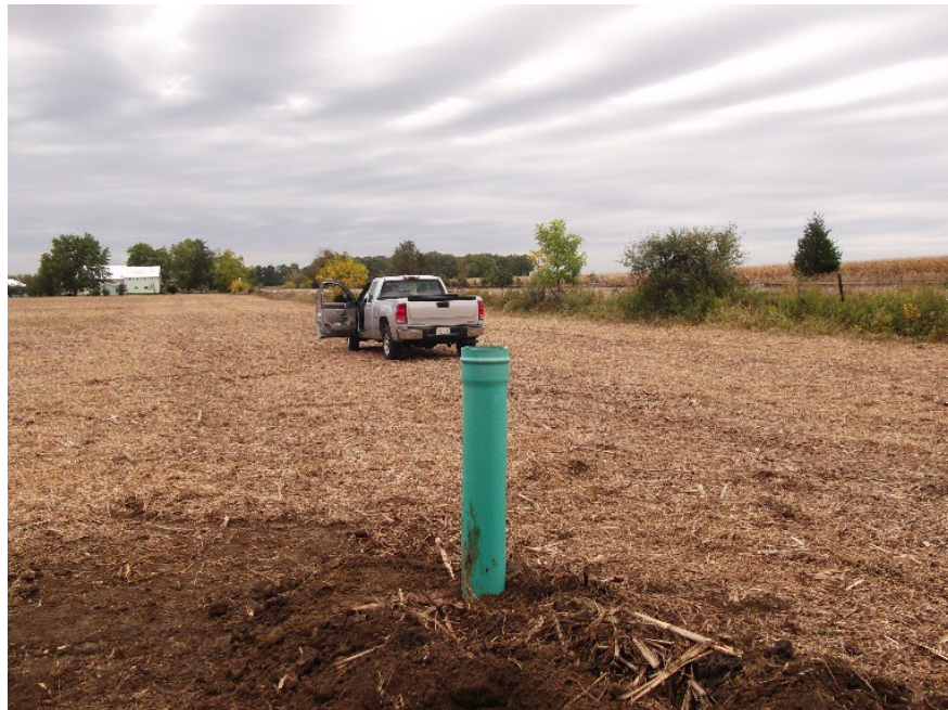
Wasson #1 wellhead after emergency work
