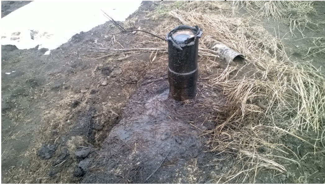
Wasson #1 well before emergency work
