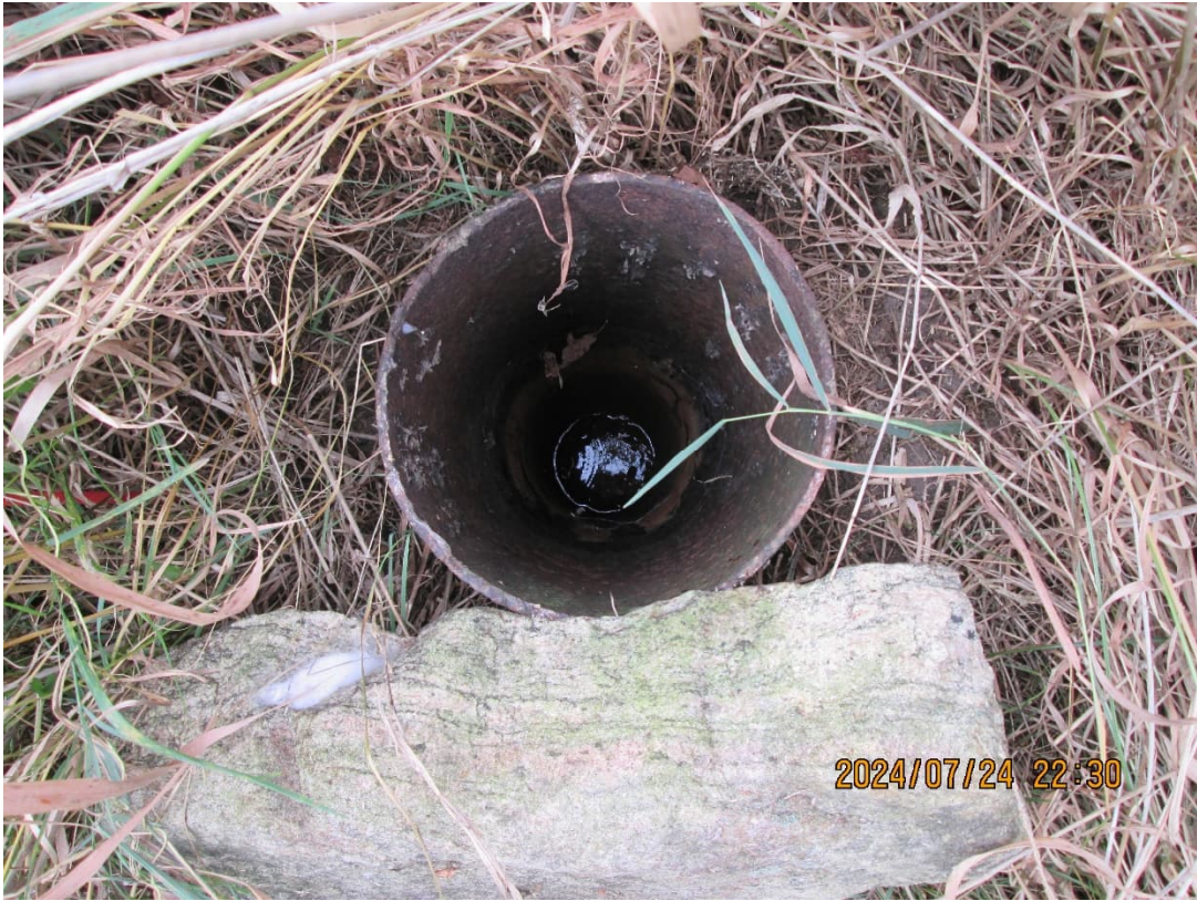
View of casing and liquid within casing.
