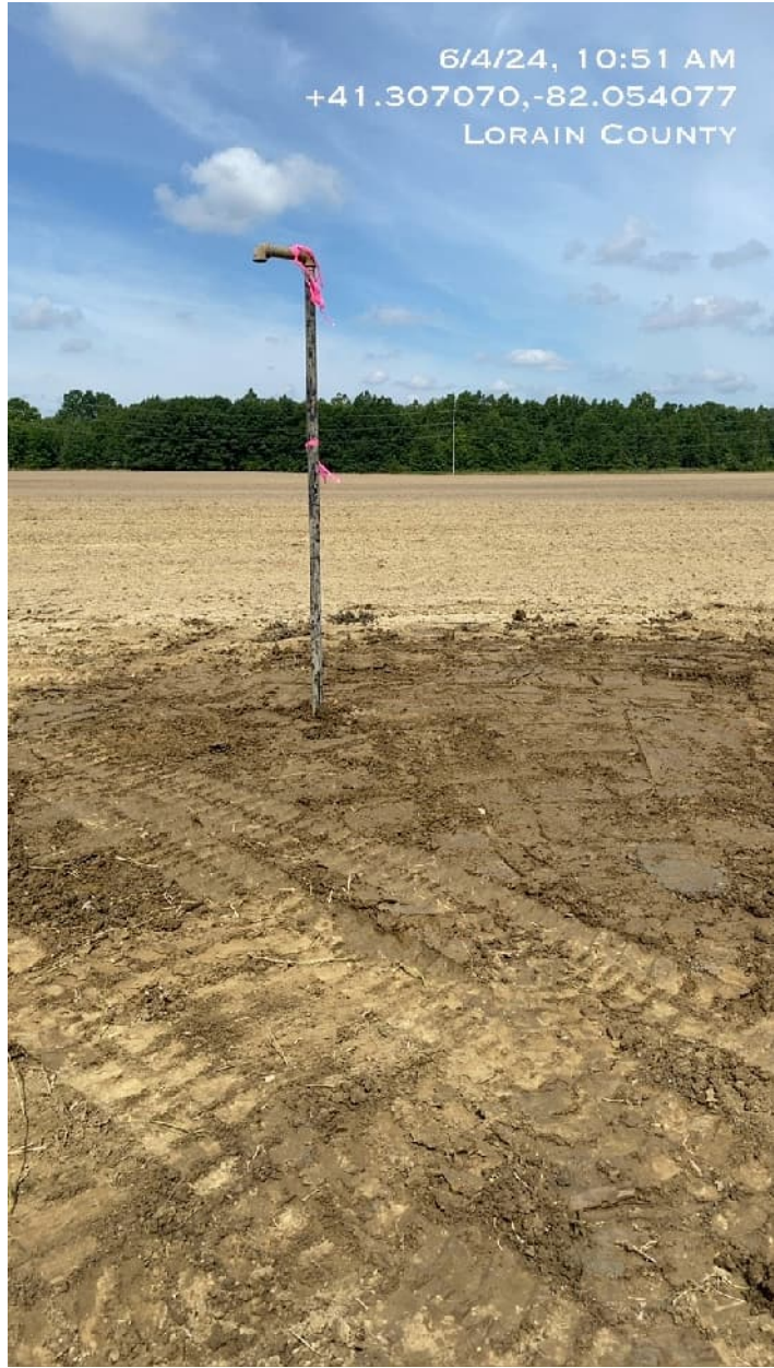
2024 photo of the Carpenter-Yost #1 showing the completed vault and vent system installed over the well.
