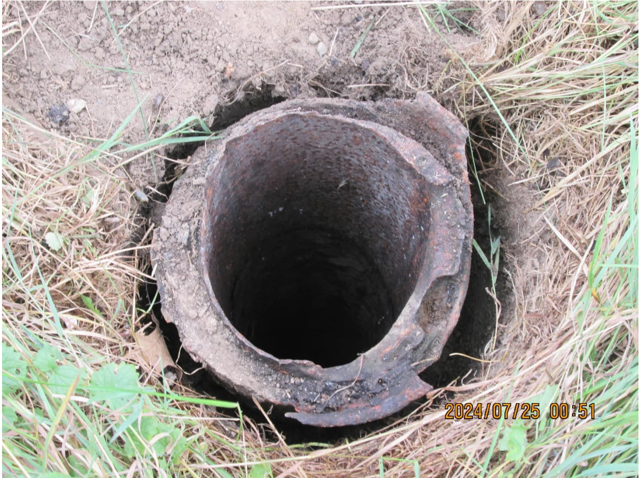
View of Midview School District #1 surface casing.
