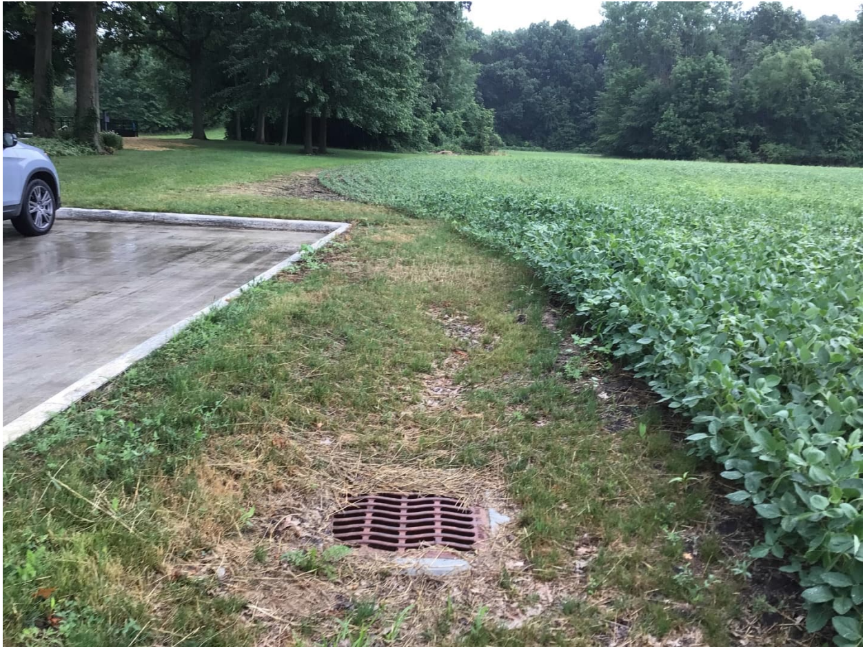
View looking northwest of access entrance and storm water inlet.
