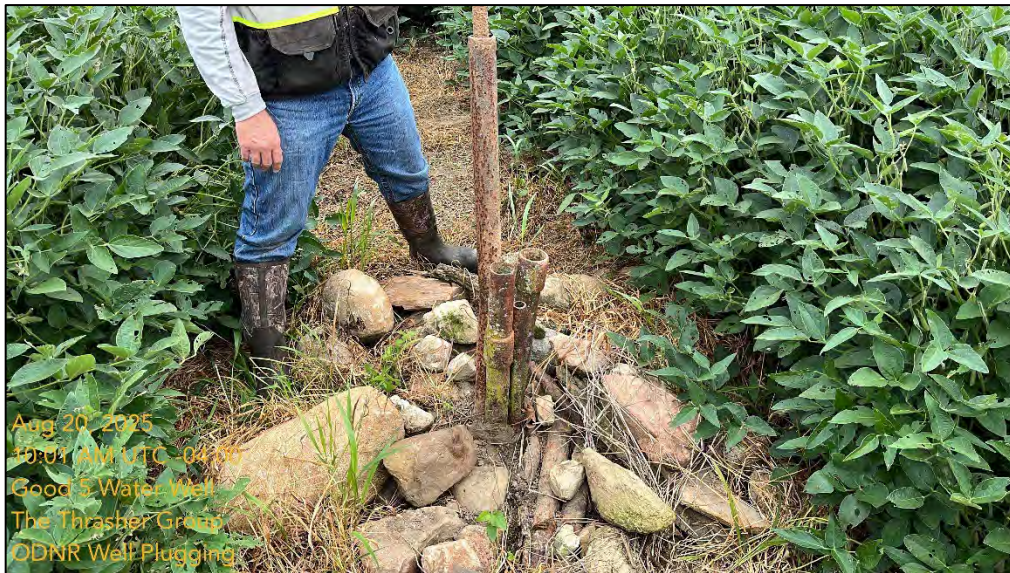
Photograph #1: Good 5 Water Well
