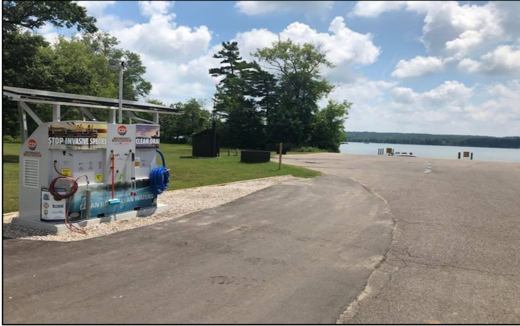
Figure 59. A public boat washing station for boat access sites.
