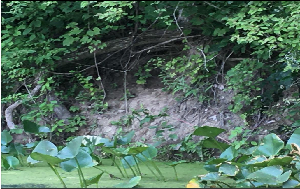
Figure 67. Shoreline erosion on an Indian Lake canal (July, 2023).
