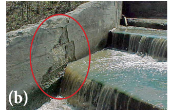
(a) The steel poles were used to hold a fish screen; the dam nearly failed during a flood because the screen collected debris and obstructed the spillway. The poles and screen were directed to be removed. (b) Spalled concrete can expose reinforcing steel, which can lead to rapid deterioration.
