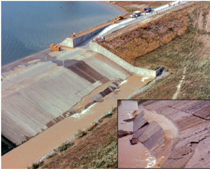
This dam is failing because of seepage under the spillway.
