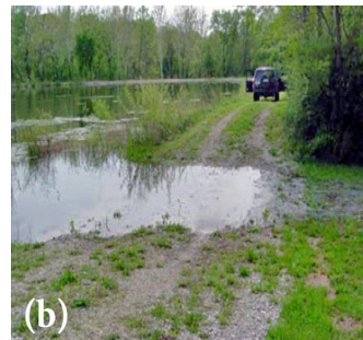
(a) Embankment crests with vehicle ruts will collect water and weaken the embankment. (b) Crest beginning to overtop in low area. This could lead to erosion and failure of the dam.
