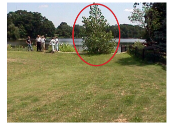
A tree is obstructing this spillway.
