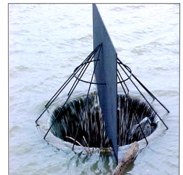
Trashracks with properly sized openings will pass smaller debris and stop larger items.
