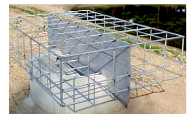
A trashrack with properly sized openings, large surface area and an anti-vortex plate will likely perform best.
