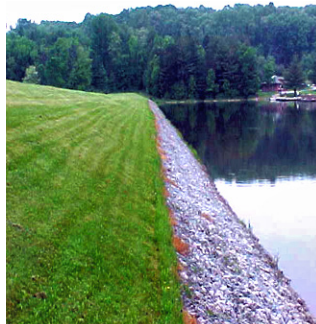
This slope is well maintained with rock riprap along the shoreline.
