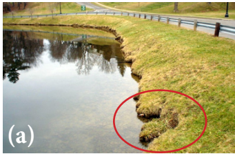
(a) Collapsed muskrat burrows increase shoreline erosion and sloughing. (b) This shoreline has eroded due to lack of proper erosion protection leading to sloughing and cracking of the slope.
