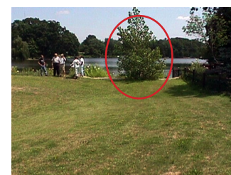
A tree is obstructing this spillway.
