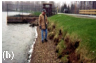
(a) Collapsed muskrat burrows increase shoreline erosion and sloughing. (b) This shoreline has eroded due to lack of proper erosion protection leading to sloughing and cracking of the slope.
