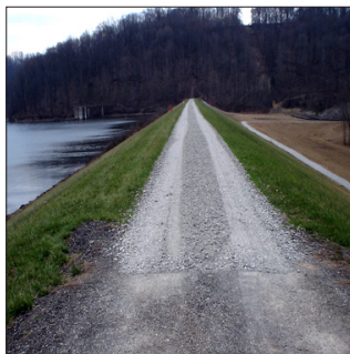
Crest with a good cover that will reduce the effects of vehicular traffic.
