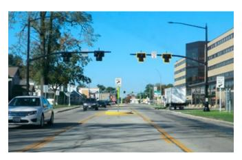
A pedestrian hybrid beacon (PHB) stops traffic so pedestrians can cross safely. The beacon, which is two red signals above a yellow one, is activated by pedestrians when they want to cross the street. First, yellow warning lights flash letting drivers know to slow down. Then there is a solid red light, telling drivers to stop so pedestrians can cross. When the beacon begins flashing red, drivers can proceed if the crosswalk is clear.
