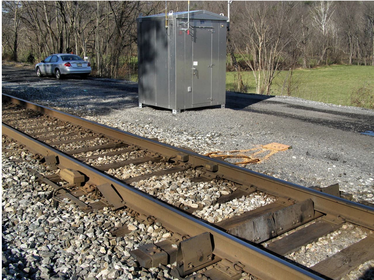
Figure 4-13. Hot Box and Dragging Equipment Detector
