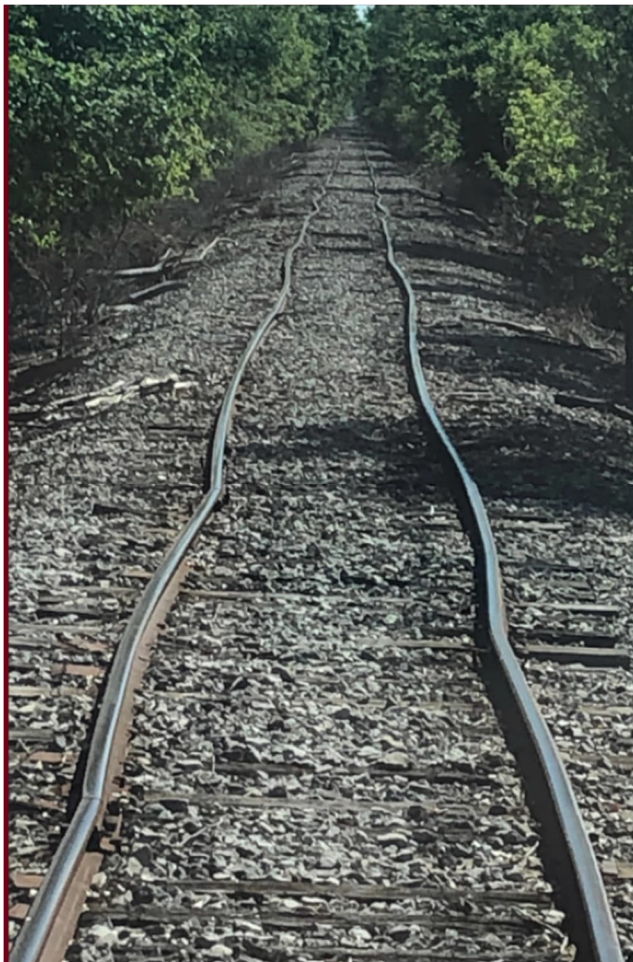
Figure 4-9. NDW Tracks before Improvements
