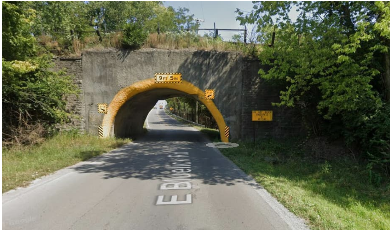
Figure 4-16. Rail Overpass in Lima Frequently Struck by Trucks
