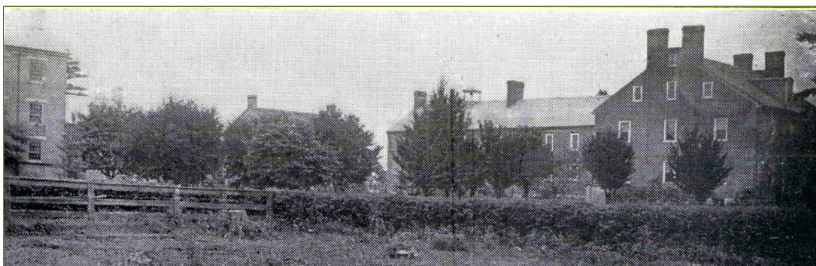
Figure 35. North Family Lot, Union Village looking southeast from curve in the road, communal house (right) and corner of Sisters' Carding Shop (left) (Phillippi 1912:96)
