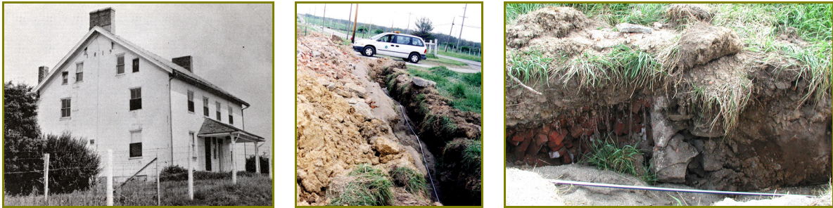
Figure 14. West Brick Family communal house, ca. 1917 (left); waterline trench through communal house basement in 2003 (center); exposed west stone foundation wall of communal house (right) (1917 West Brick house: Otterbein Homes Museum and Library archives; 2003 trench: ODOT project file)
