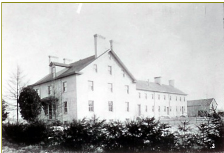
Figure 50. Ca. 1890 Center Brick House, Center Family Lot, Union Village (South Union Village Museum and Library)
