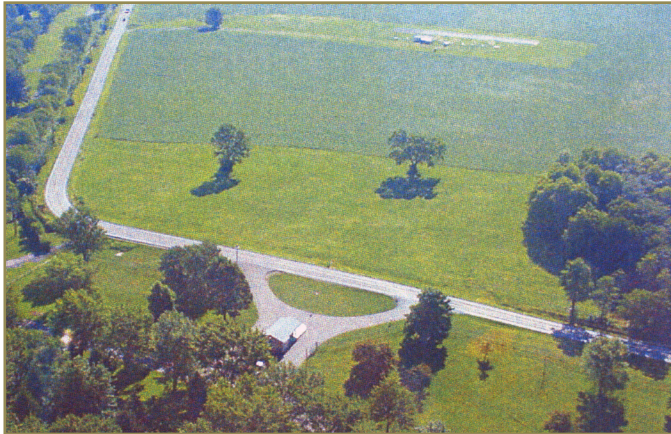
Figure 1. Overview in 2005 of the SR 741 Curve, prior to the realignment North is toward the upper left corner. (Photograph by ODOT-Aerial Engineering)
