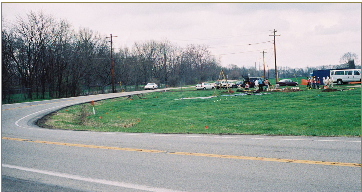
Figure 4. Overview of sharp-angled curve at the beginning of fieldwork, looking northeast
