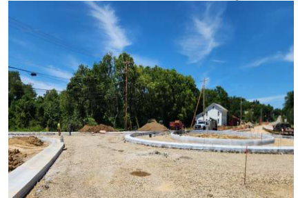
Village of Granville Roundabout - SR 661 & New Burg Street
