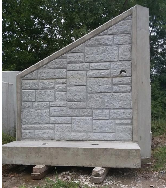
Figure 4: Wingwall With Stone Pattern
