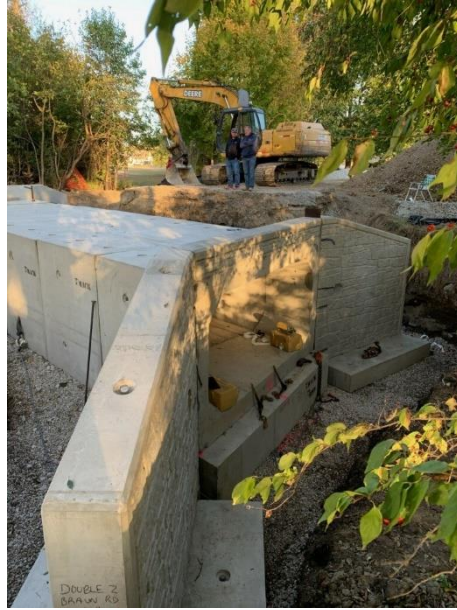
Figure 2: Installed Wingwalls At Braun Rd. PID No. MAD-TR232-1.02
