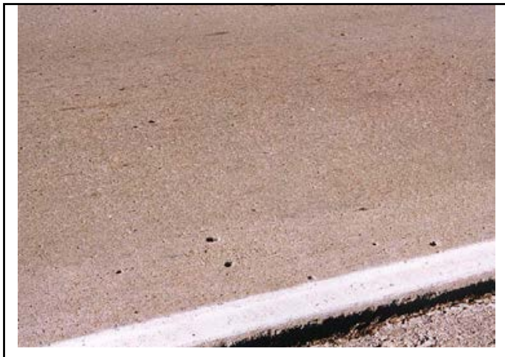
Photo D-4. Popouts in CRC Pavement
