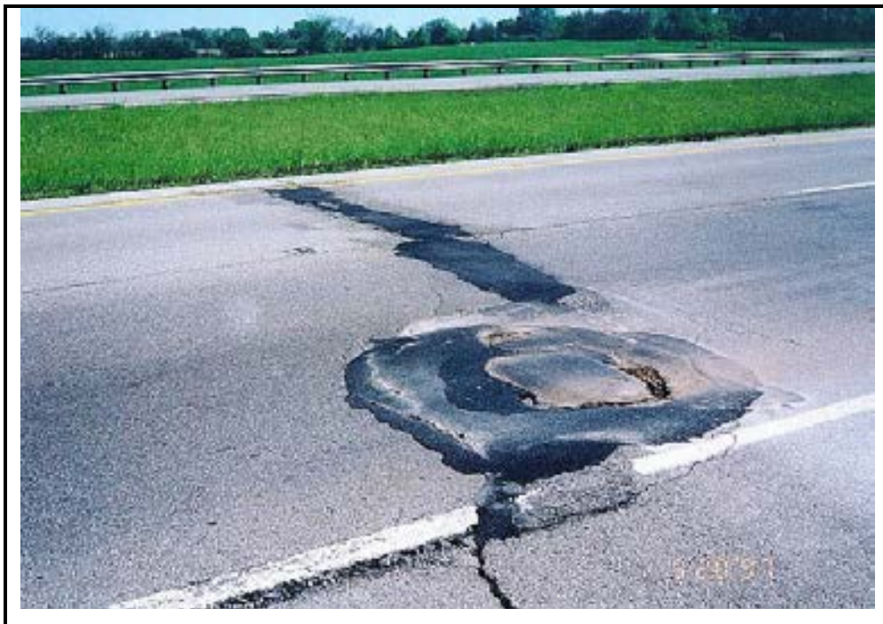
Photo B-12. Pumping in Composite Pavement
