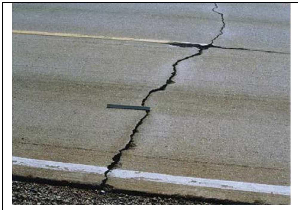
Photo C-9. Faulting in Jointed Concrete Pavement
