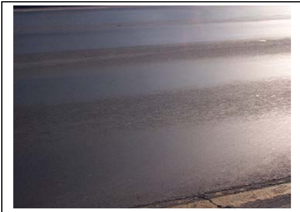
Photo E-4. Bleeding in Local Pavement, High Severity High Severity shows most aggregates covered with asphalt.
