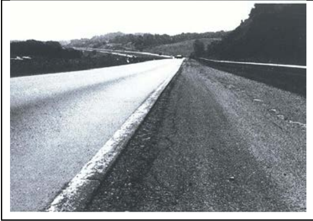
Photo D-9. Settlement in CRC Pavement
