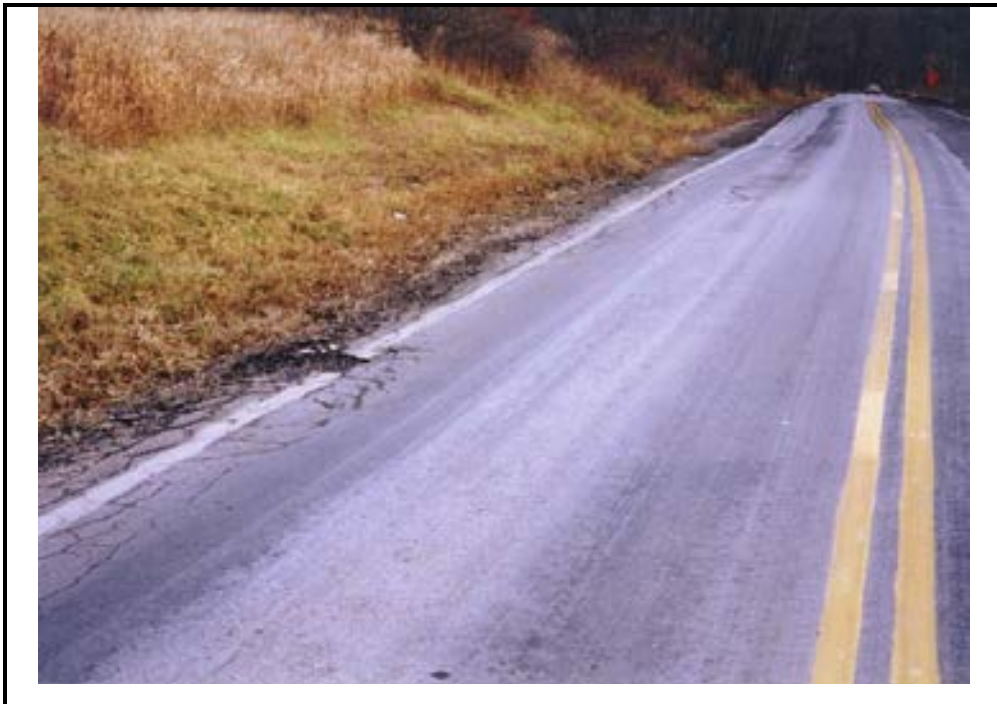
Photo A-22. Edge Cracking in Flexible Pavement, High Severity
