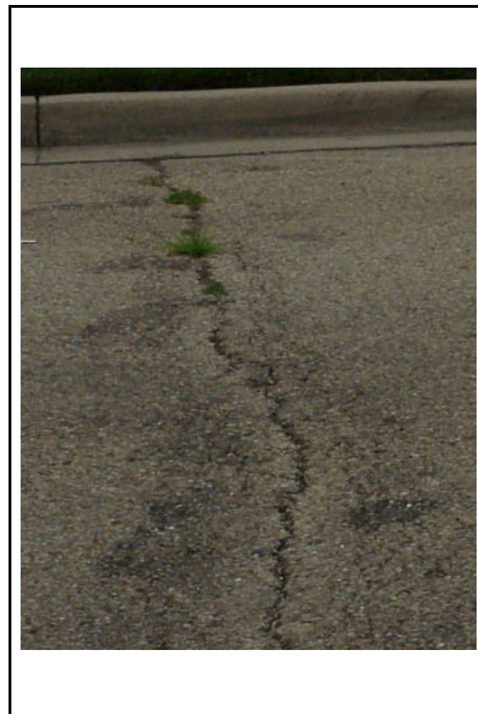
Photo E-17. Transverse Cracking in Local Pavement, High Severity
