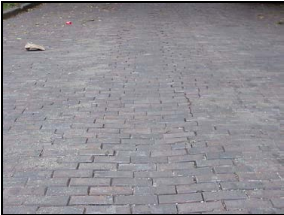
Photo F-10. Rutting in Brick Pavers, Low Severity
