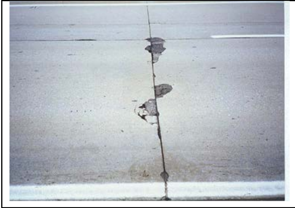
Photo C-4. Patching in Jointed Concrete Pavement, Low Severity
