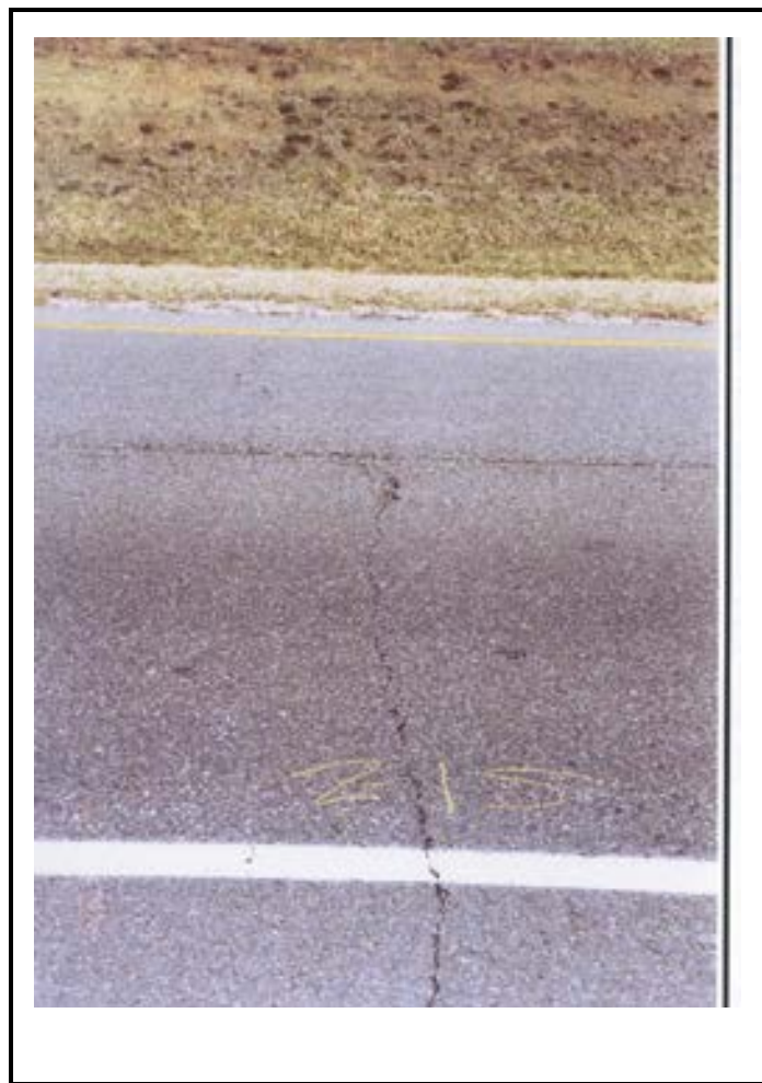
Photo B-15. Unjointed Base, Transverse Cracking in Composite Pavement, Low Severity
