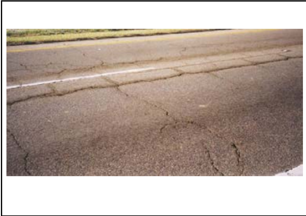
Photo A-8. Crack Sealing Deficiency in Flexible Pavement, Unsealed Cracks
