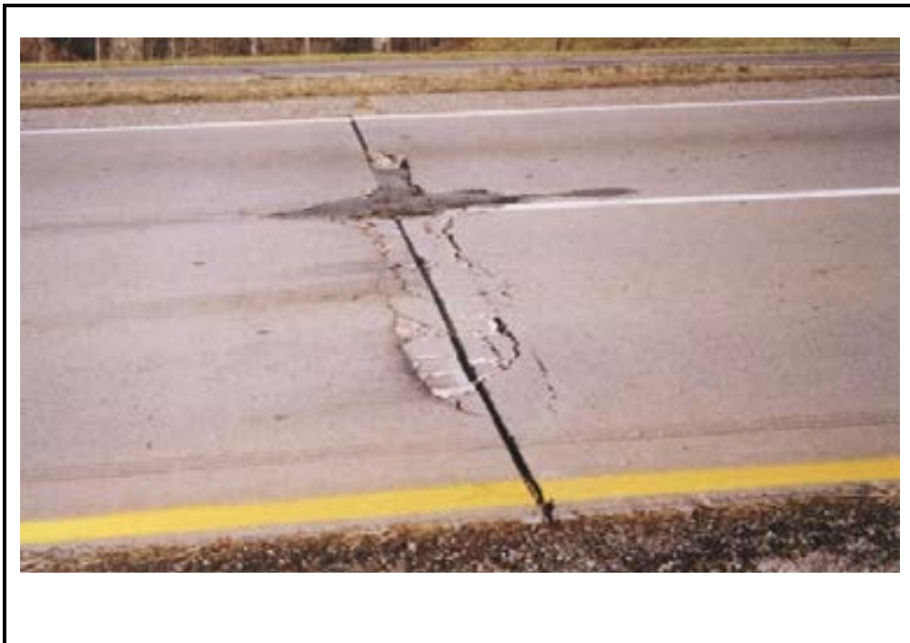
Photo C-12. Transverse Joint Spalling in Jointed Concrete Pavement, High Severity
