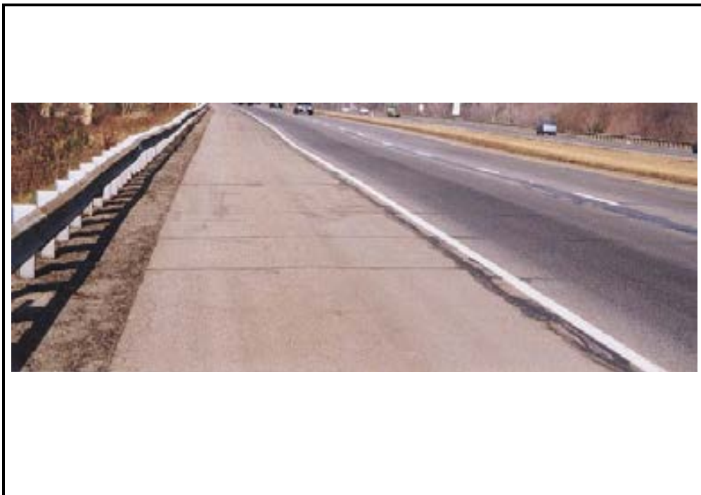
Photo A-13. Settlement in Flexible Pavement, Medium Severity
