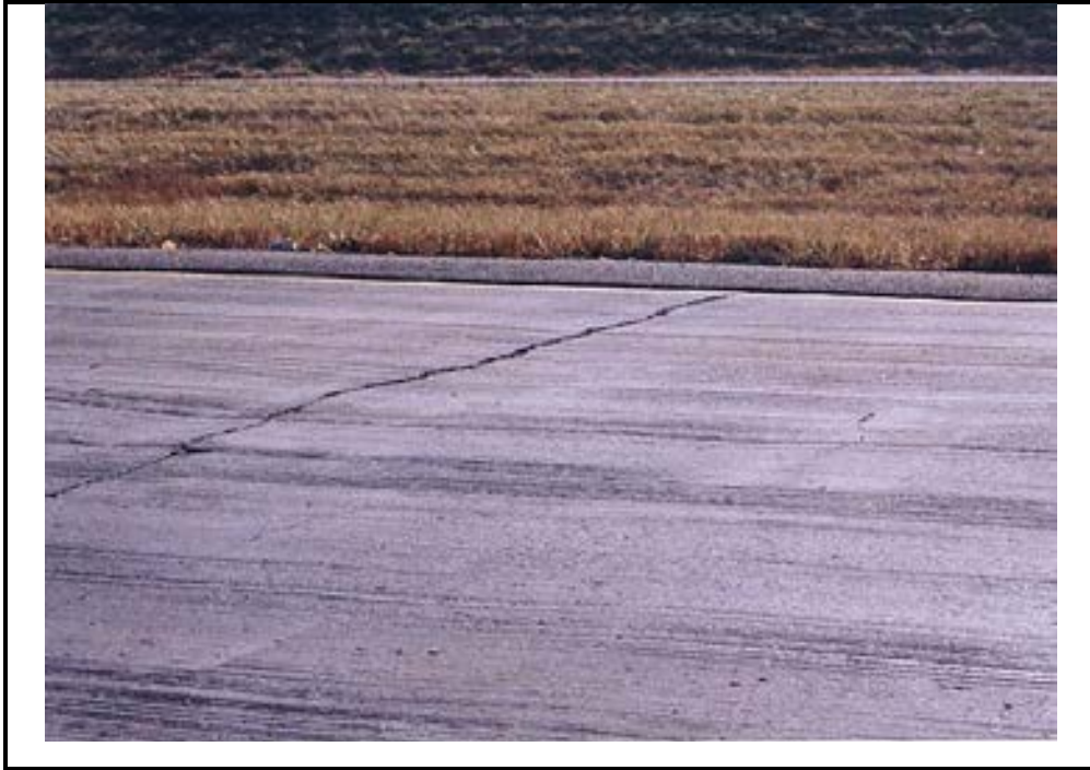
Photo D-10. Transverse Cracks in CRC Pavement, Low Severity
