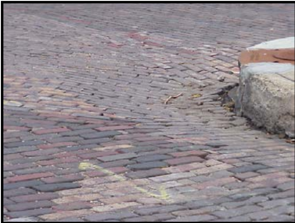
Photo F-16. Settlement in Brick Pavers, High Severity
