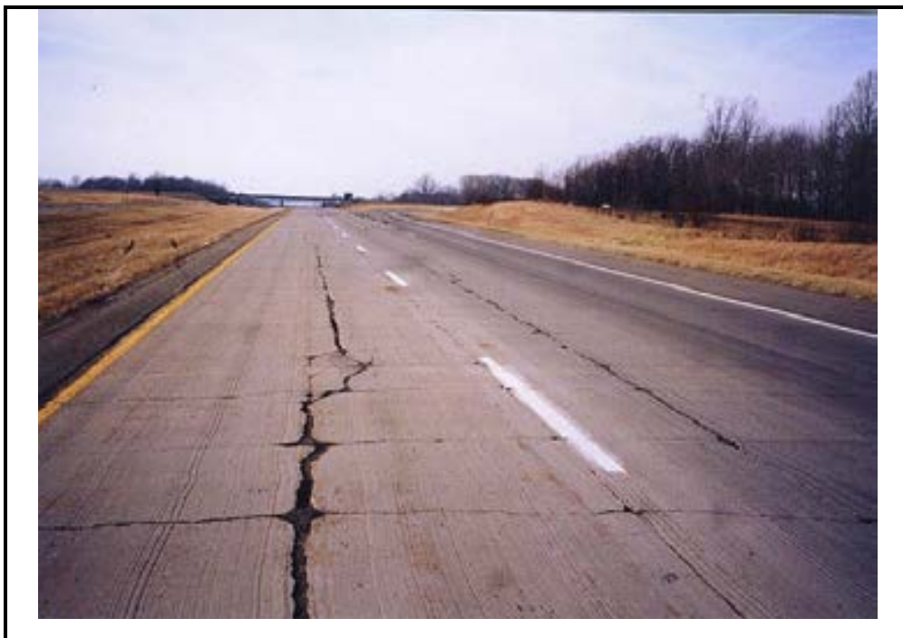
Photo D-13. Longitudinal Cracking in CRC Pavement, High Severity
