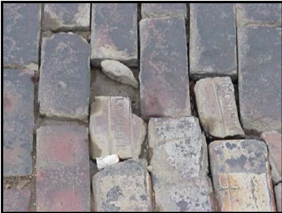
Photo F-14. Joint Erosion in Brick Pavers, High Severity
