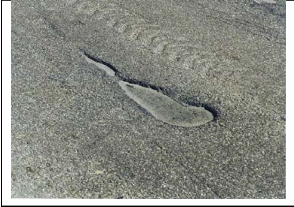
Photo A-7. Debonding in Flexible Pavement, Medium Severity
