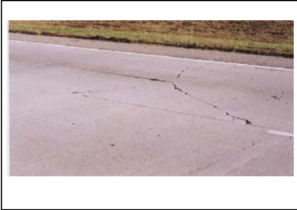
Photo C-18. Longitudinal Cracking in Jointed Concrete Pavement, Medium Severity
