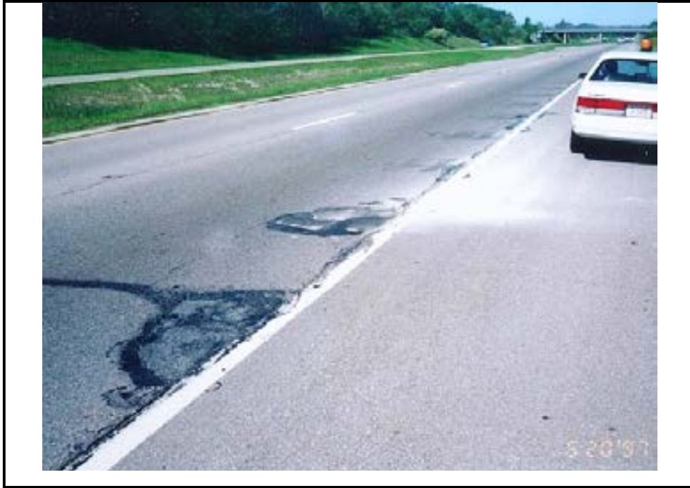
Photo B-11. Pumping in Composite Pavement
