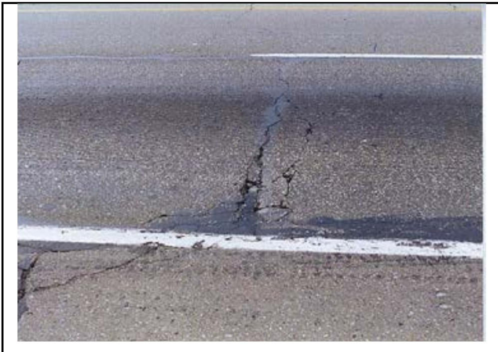
Photo A-9. Crack sealing Deficiency in Flexible Pavement, Cracks not sealed properly
