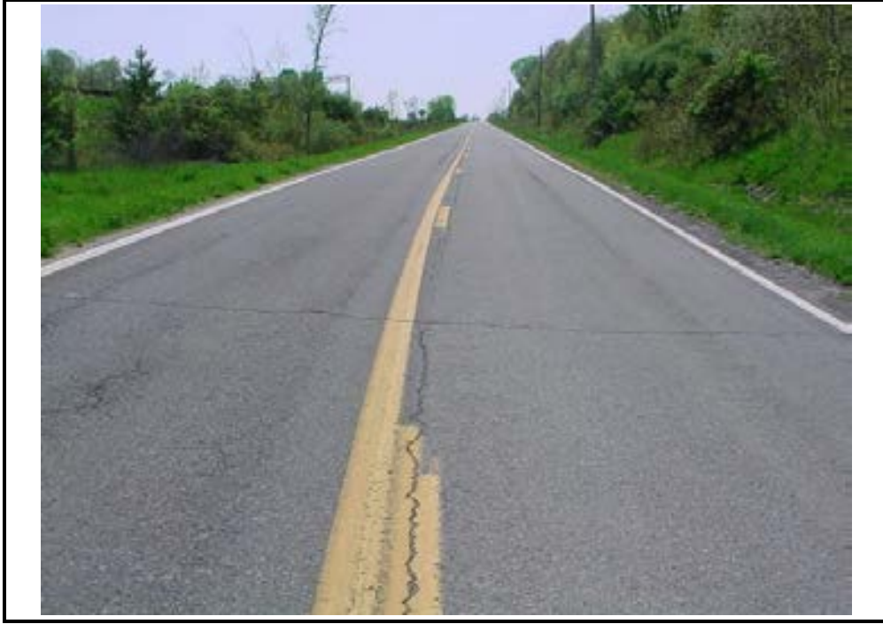
Photo A-23. Thermal Cracking in Flexible Pavement, High Severity
