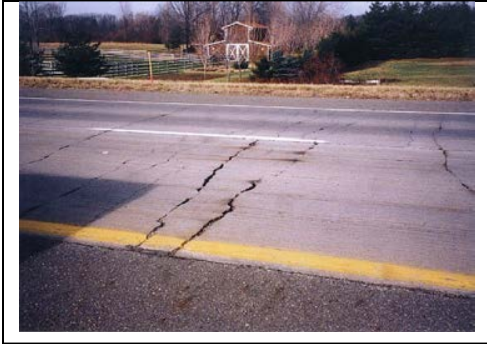
Photo D-16. Spalling in CRC Pavement, Medium Severity
