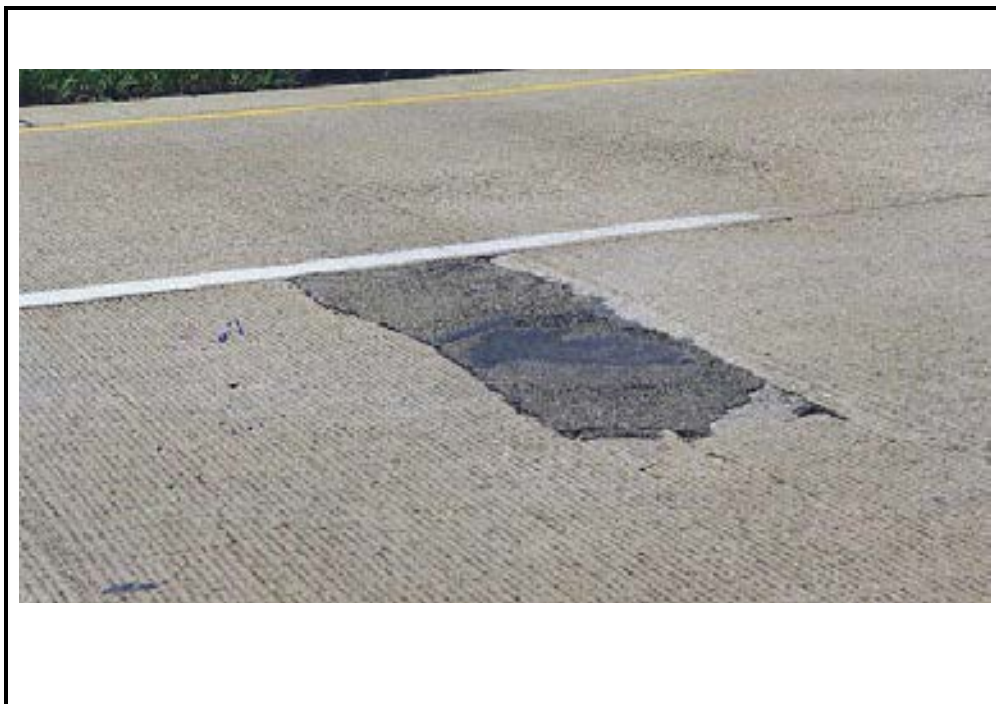
Photo C-5. Patching in Jointed Concrete Pavement, High Severity
