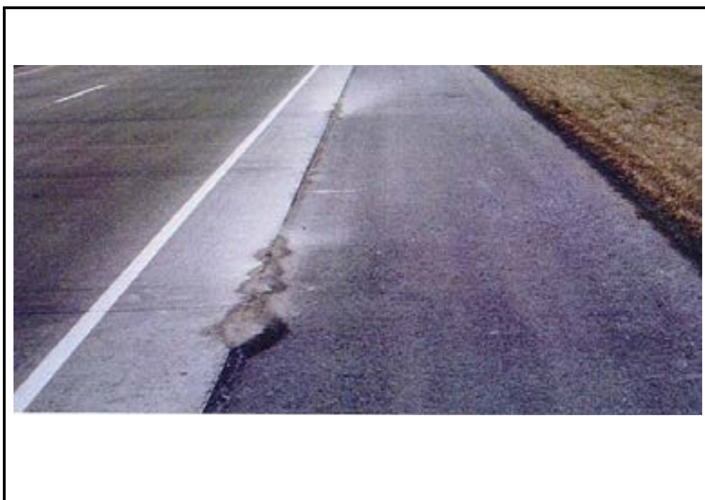
Photo C-7. Pumping in Jointed Concrete Pavement, Low Severity
