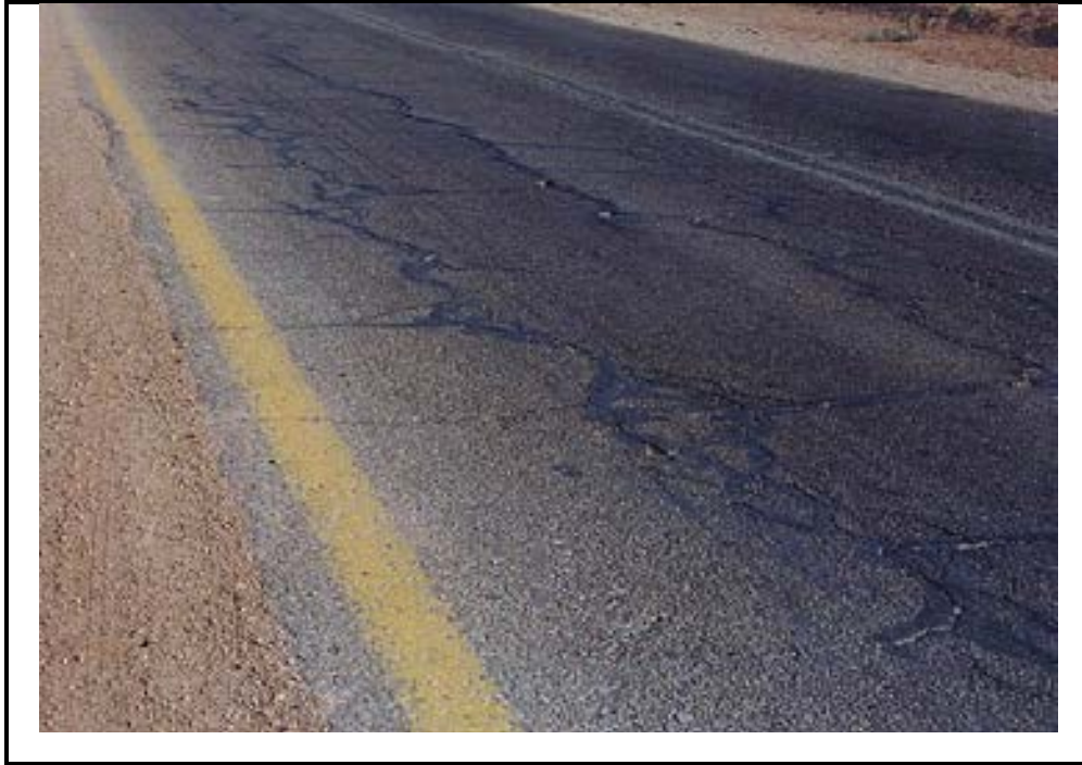
Photo A-15. Wheel Track Cracking in Flexible Pavement, Med. Severity
