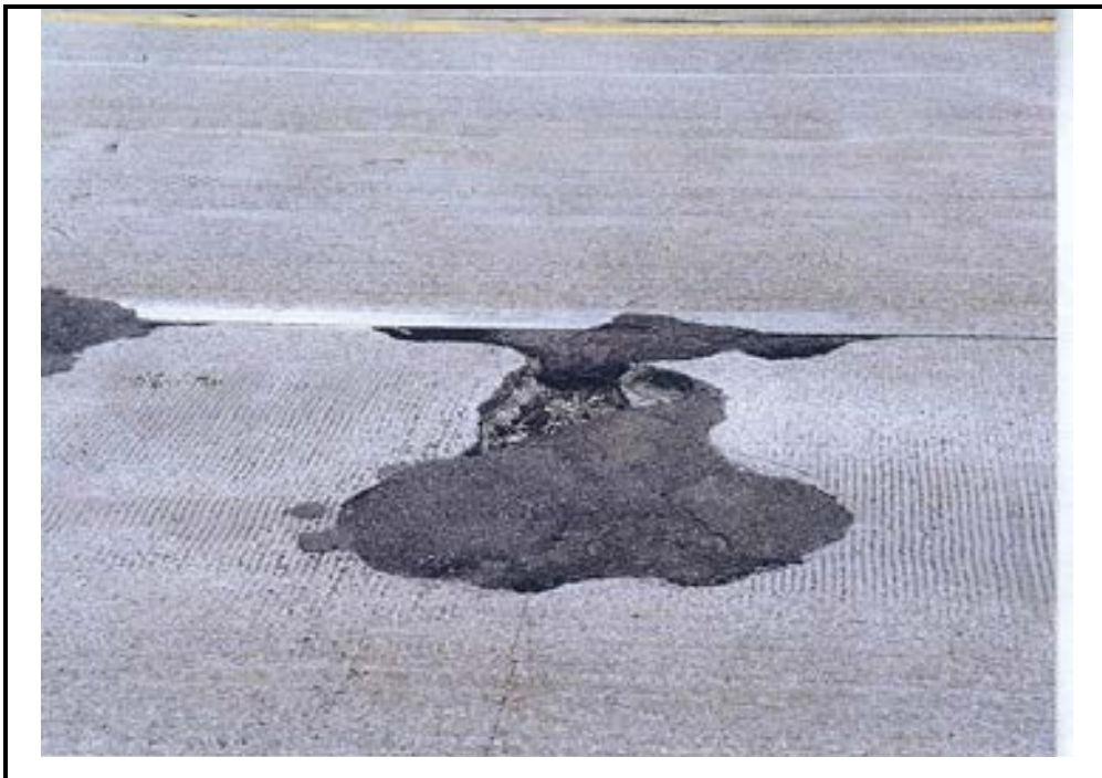
Photo D-6. Patching in CRC Pavement, High Severity
