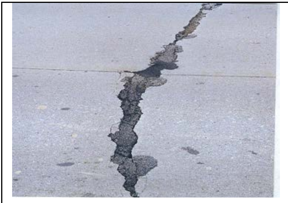
Photo D-17. Spalling in CRC Pavement, High Severity
