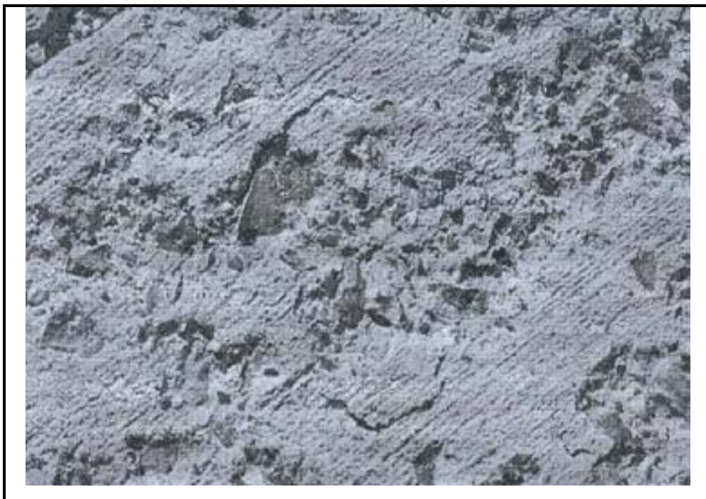
Photo D-2. Surface Deterioration in CRC Pavement, High Severity
