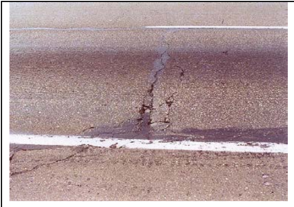
Photo B-22. Crack Sealing Deficiency in Composite Pavement, Cracks not sealed properly
