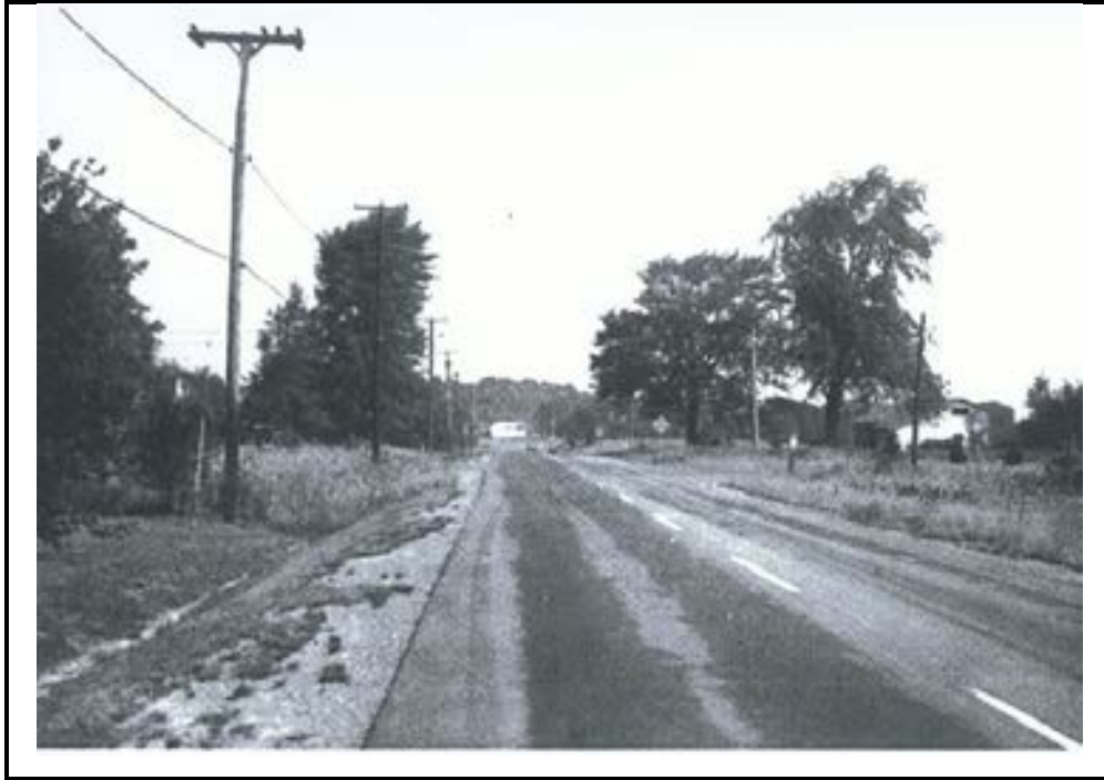
Photo B-3. Bleeding in Composite Pavement, High Severity
