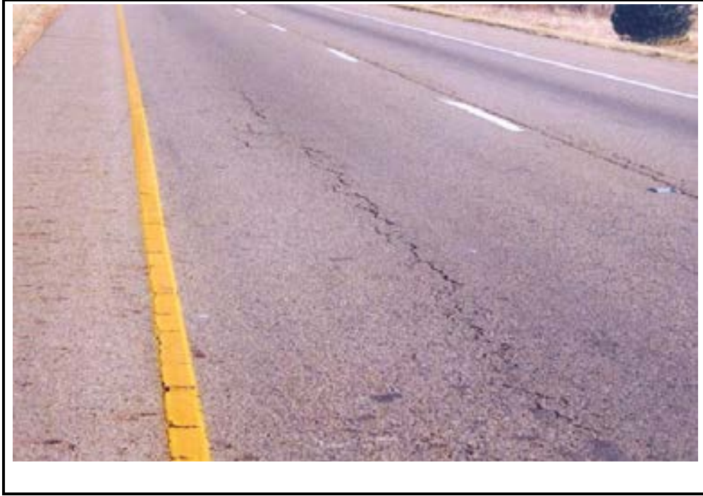
Photo A-19. Longitudinal Joint Cracking in Flexible Pavement, Medium Severity
