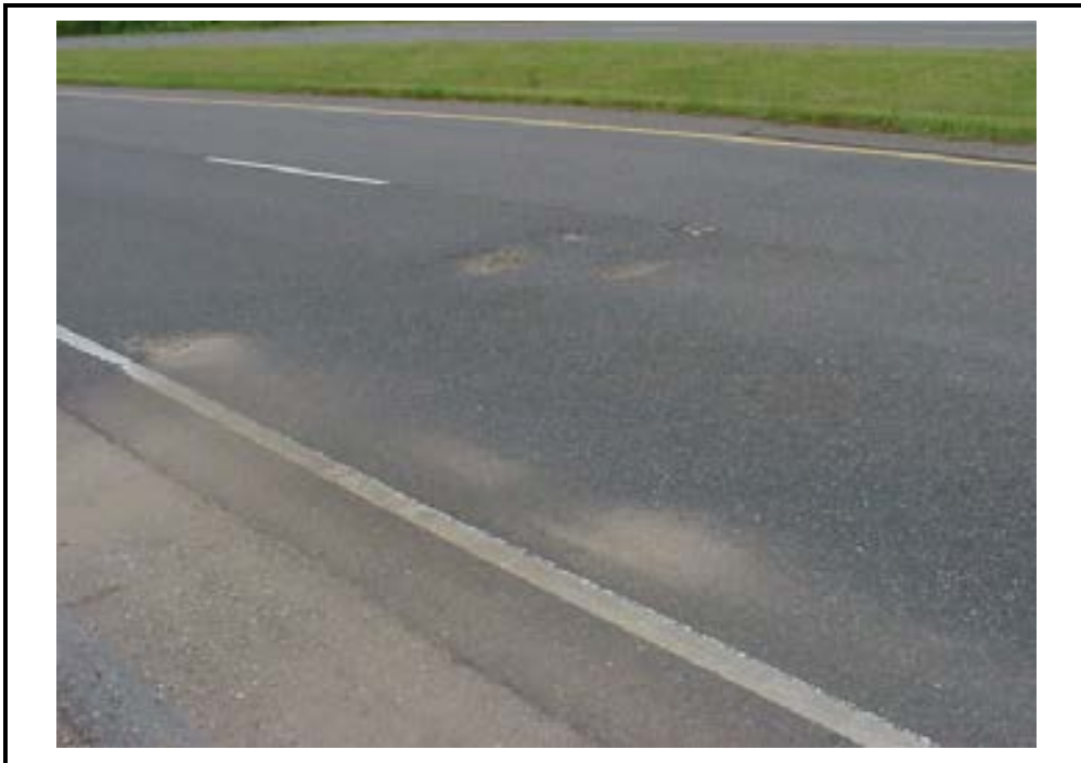
Photo B-25. Punchouts in Composite Pavement, Medium Severity
