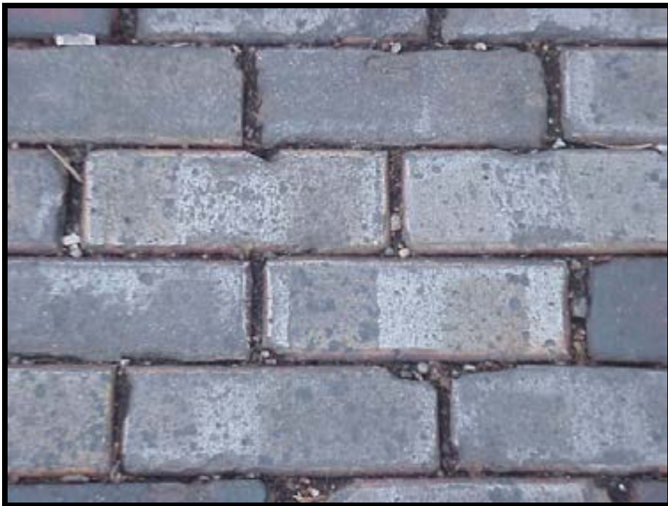
Photo F-4. Discoloration on Brick Pavers
