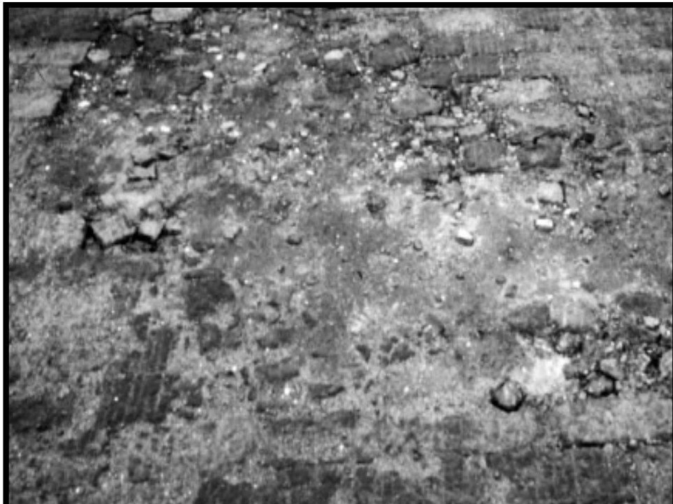
Photo F-2. Brick Deterioration in Brick Pavers, High Severity
