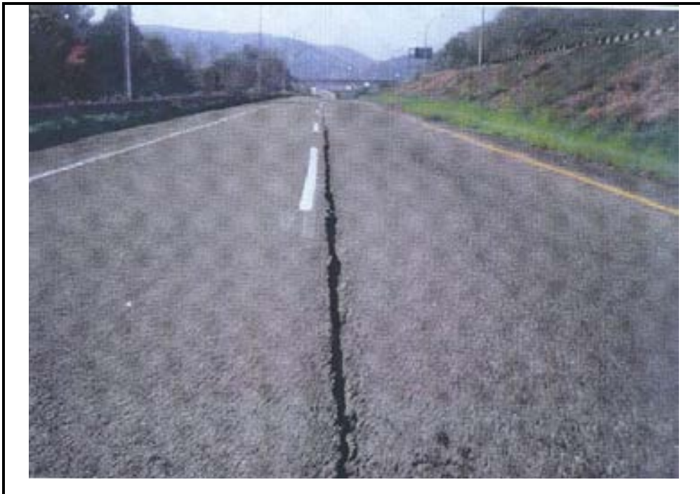
Photo A-20. Longitudinal Joint Cracking in Flexible Pavement, High Severity
