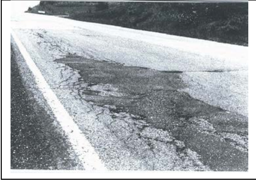
Photo A-5. Patching in Flexible Pavement, High Severity
