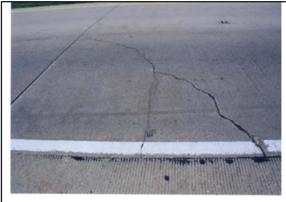
Photo C-21. Corner Breaks in Jointed Concrete Pavement, High Severity
