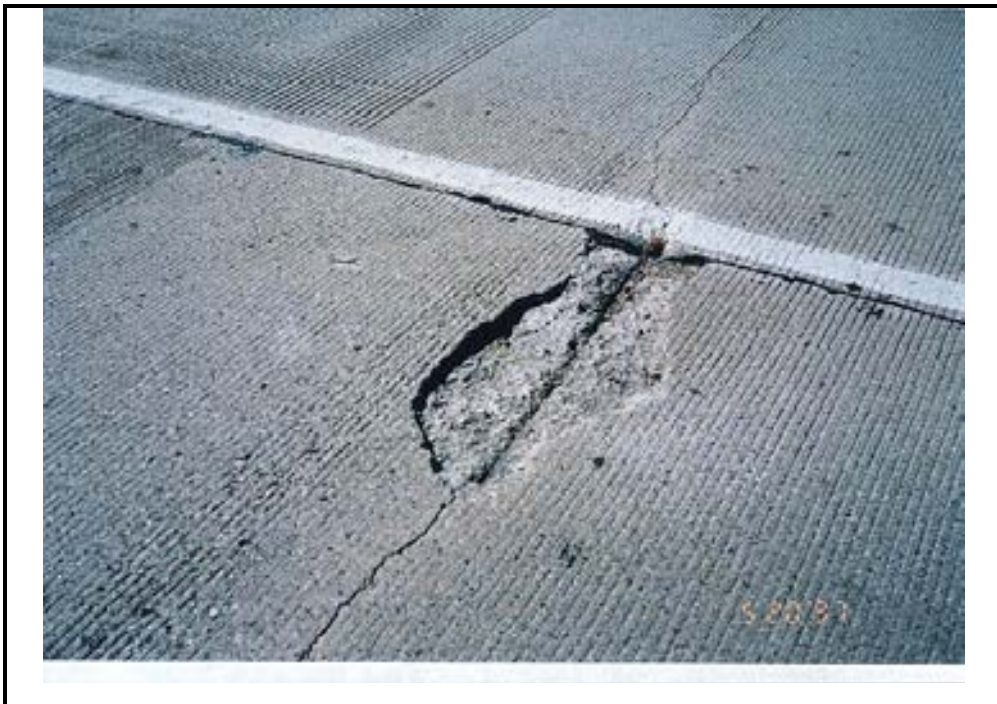
Photo C-15. Pressure Damage in Jointed Concrete Pavement
