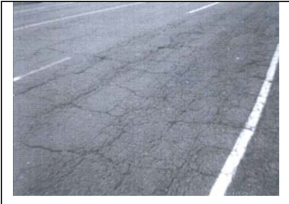
Photo A-18. Block and Transverse Cracking in Flexible Pavement, High Severity
