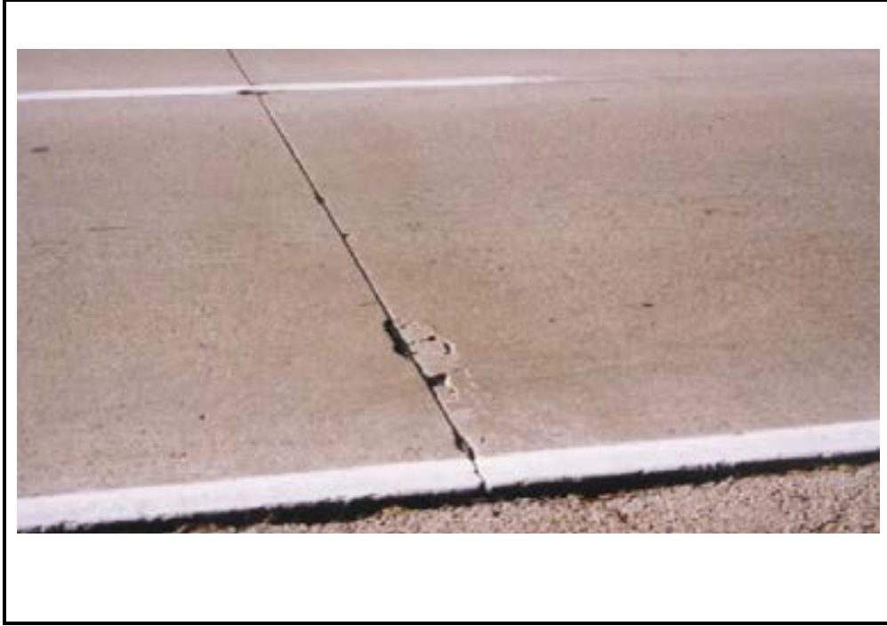
Photo C-11. Transverse Joint Spalling in Jointed Concrete Pavement, Low Severity
