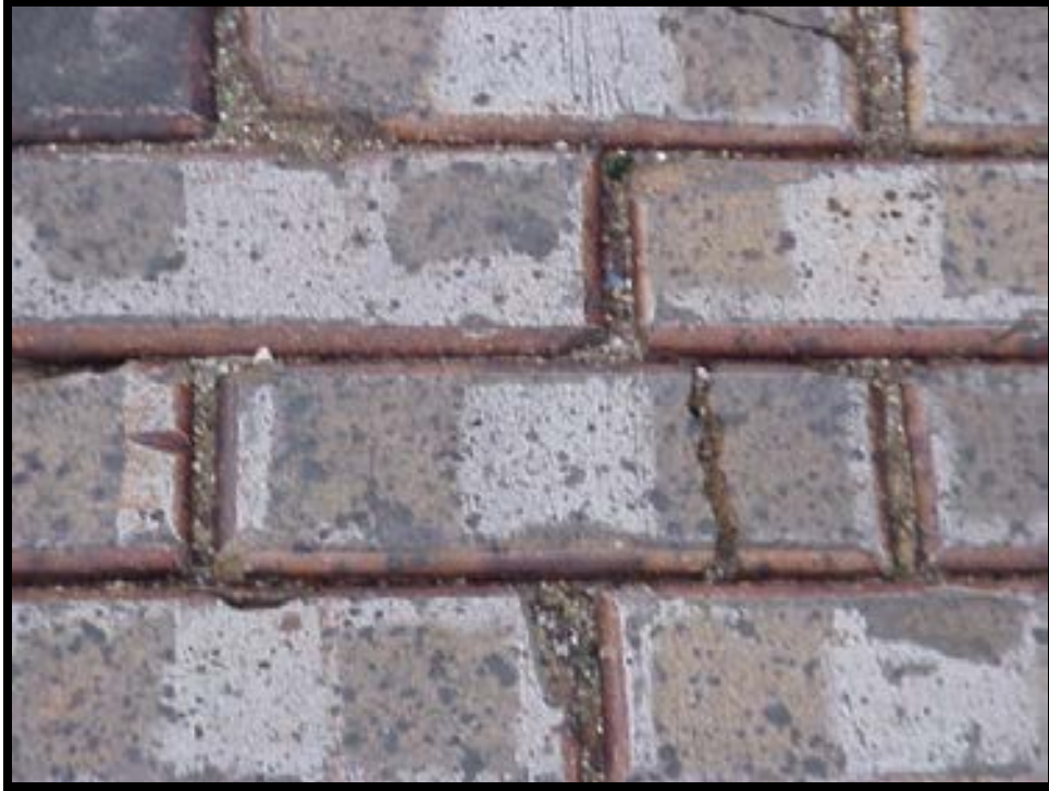
Photo F-3. Discoloration on Brick Pavers
