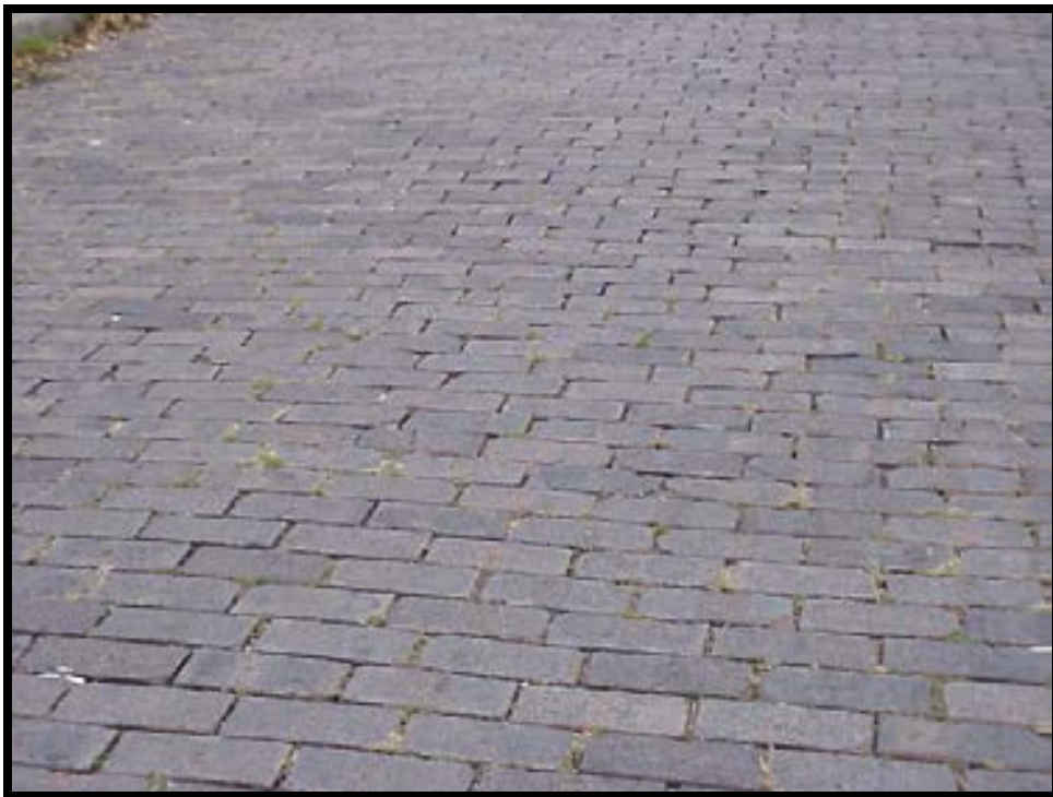
Photo F-12. Corrugations in Brick Pavers, Low Severity
