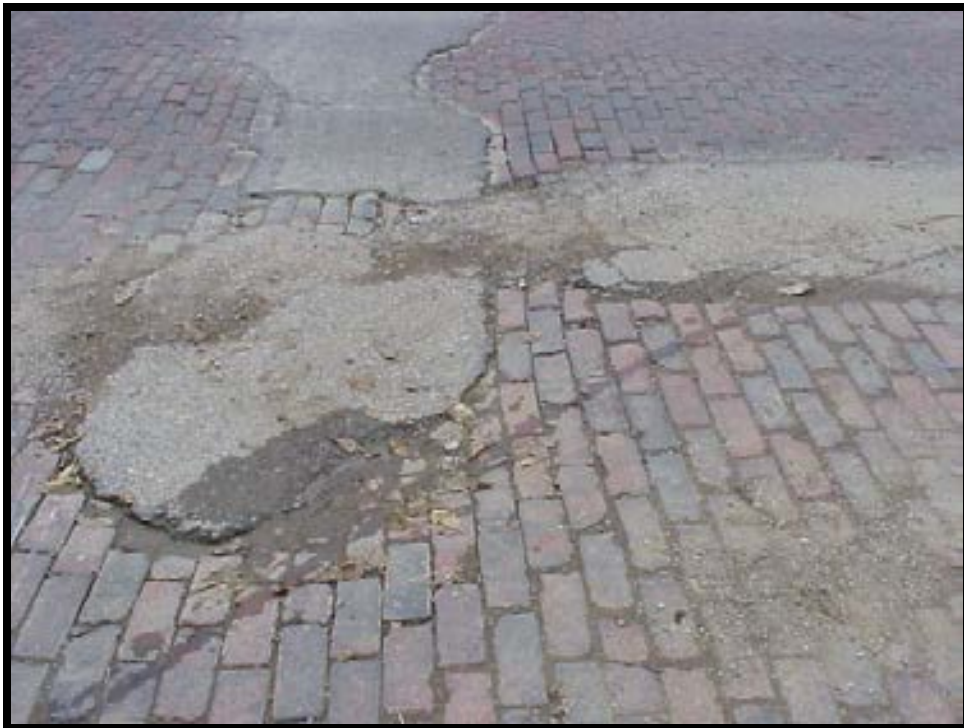
Photo F-8. Pumping in Brick Pavers
