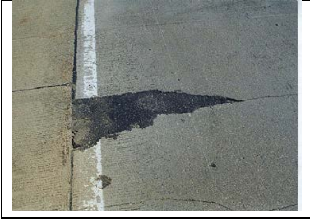
Photo D-7. Pumping in CRC Pavement, Medium Severity
