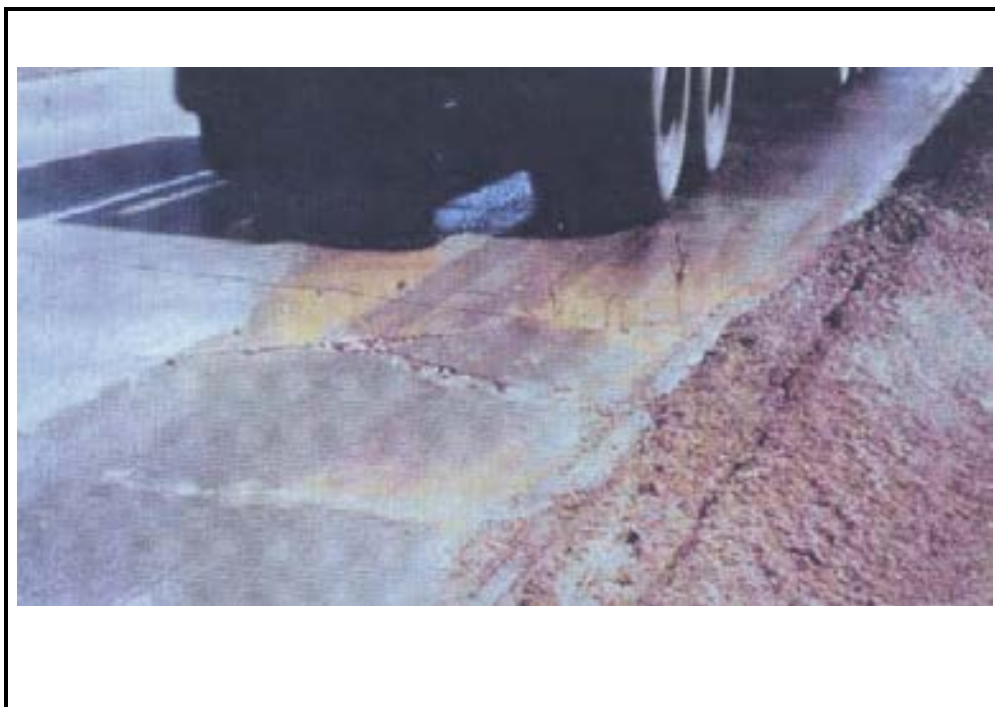
Photo C-6. Pumping in Jointed Concrete Pavement, High Severity
