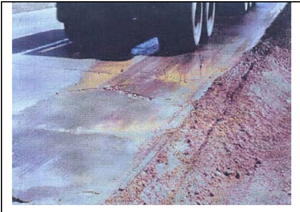
Photo D-8. Pumping in CRC Pavement, High Severity
