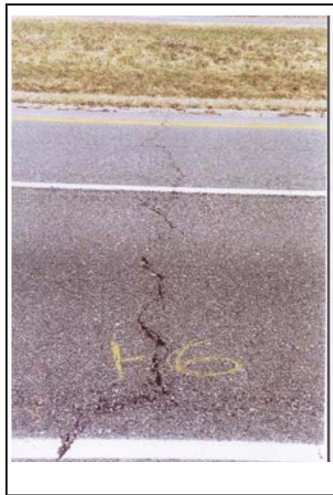
Photo B-16. Unjointed Base, Transverse Cracking in Composite Pavement, High Severity
