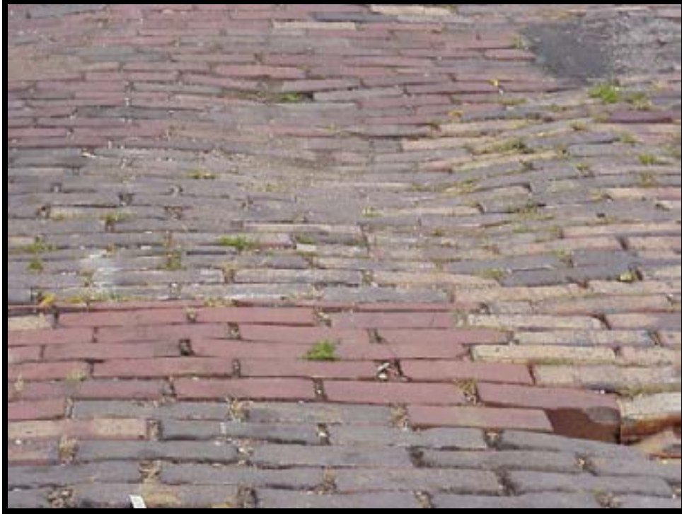
Photo F-7. Pumping in Brick Pavers
