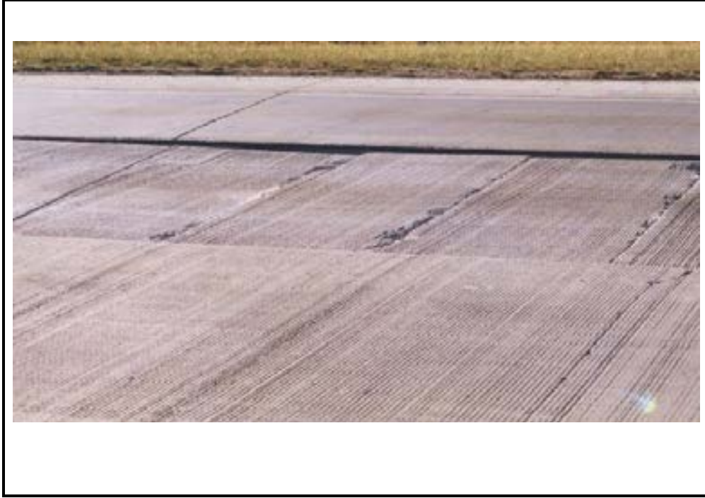
Photo C-10. Settlements in Jointed Concrete Pavement, Medium Severity
