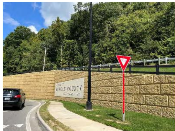
A roundabout in Morgan County.
