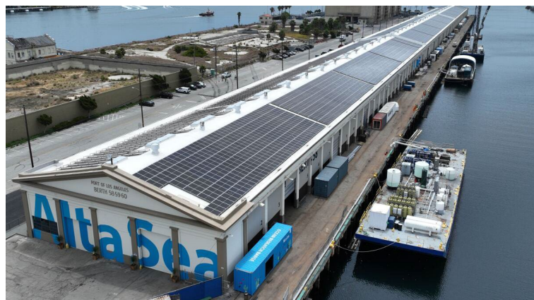
Figure 7: Port of Los Angeles Solar Panel Installation
