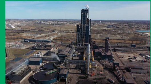
Cleveland Cliffs Direct Reduction Plant
