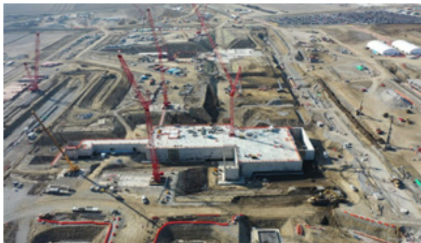
Figure 54: Construction Progress at Intel's New Albany, Ohio Site
