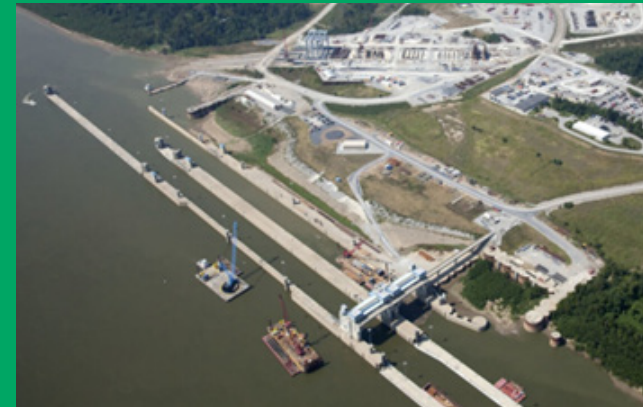
Olmsted Lock and Dam
