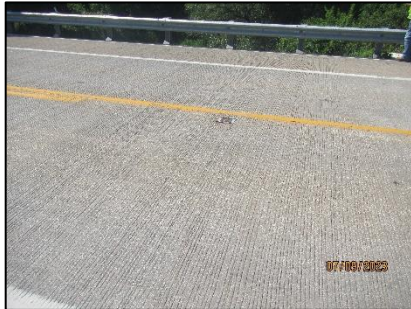
Figure 7-154: Typical wearing surface (Item B.C.01.01 – 7, Good Condition)
