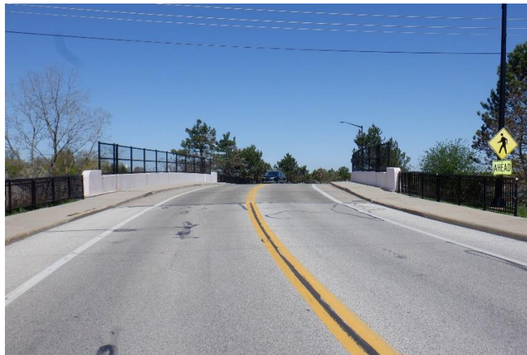
Photo 6 – Approach view to SFN 7767919, looking north.
