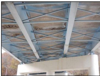
Figure 7-152: Underside of deck in Span 2
