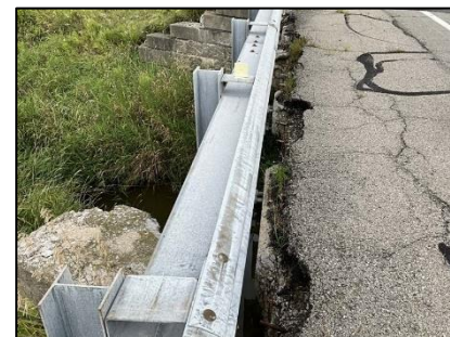
Figure 7-275: Top of deck along the right edge
