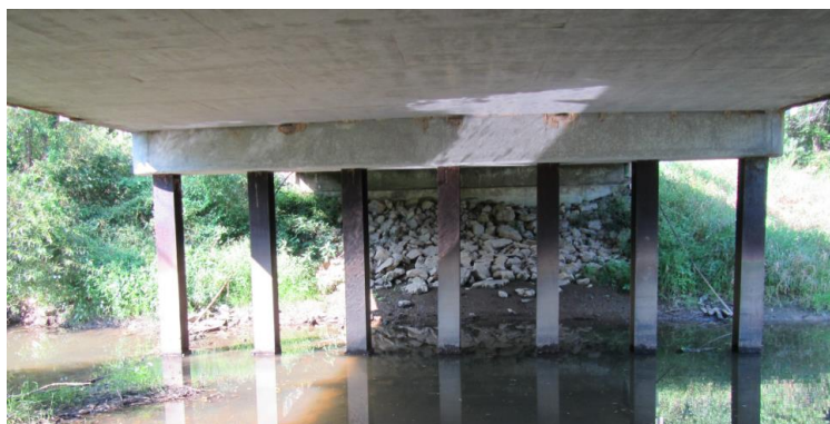
Figure 7-8: H-pile with reinforced concrete cap example.
