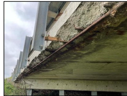
Figure 7-265: Underside of slab along the right edge
