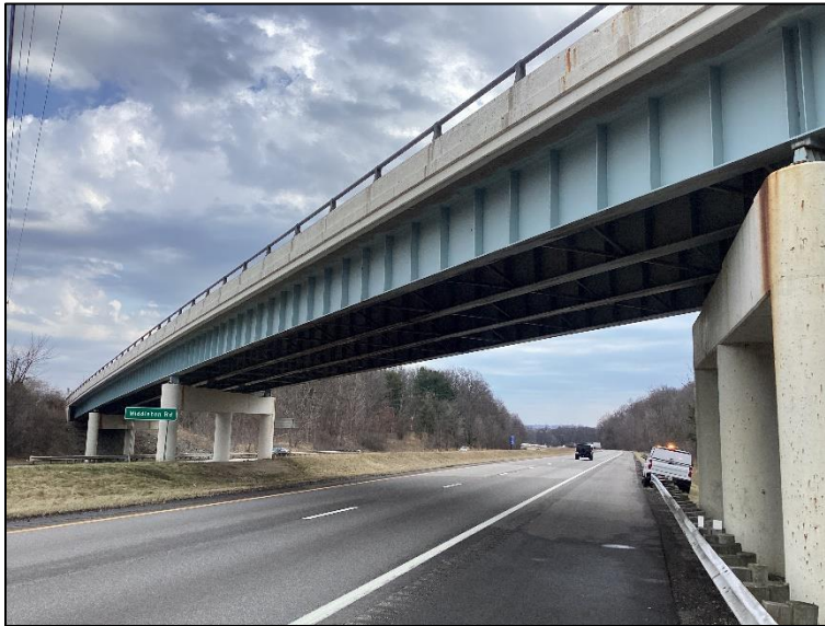
Photo 3 – Elevation view of SFN 7710569, looking northwest.
