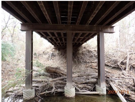
Figure 7-318: Steel intermediate pile bent.
