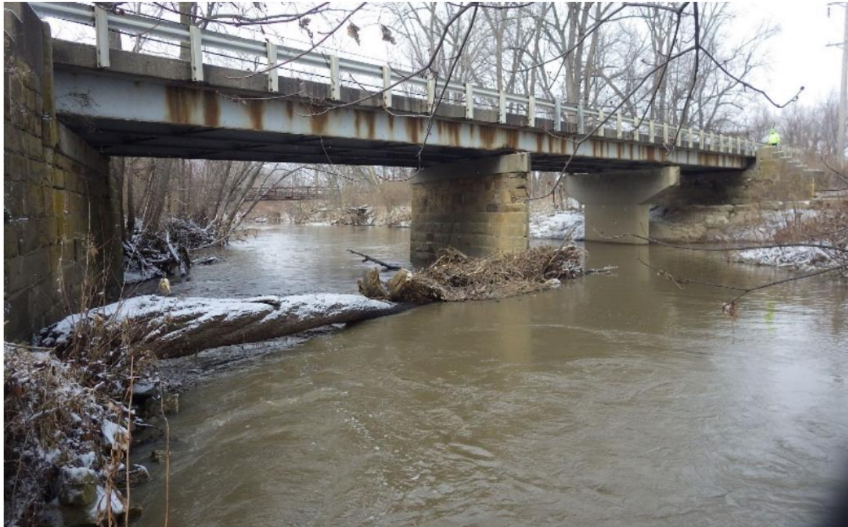
Figure 8 – Good Example of Baseline Photo Looking Downstream from SE Corner (Best Downstream Option)
