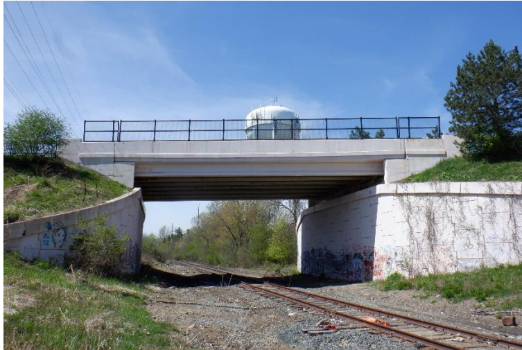
Photo 5 – Elevation view of SFN 7767919, looking west.
