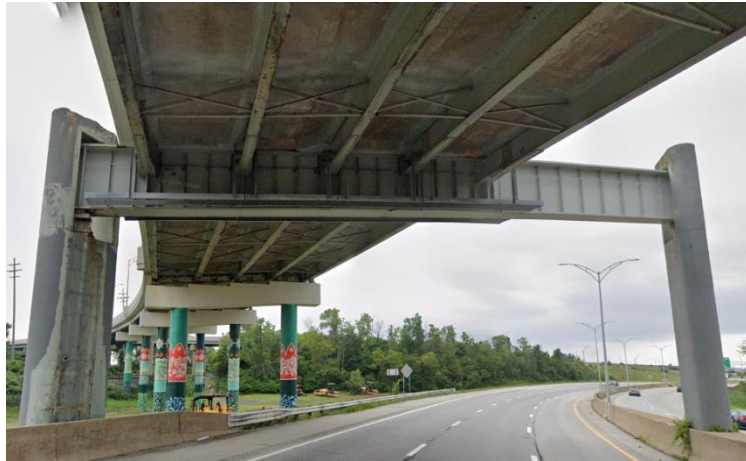
Figure 7-11: Steel straddle bent supported by reinforced concrete columns.
