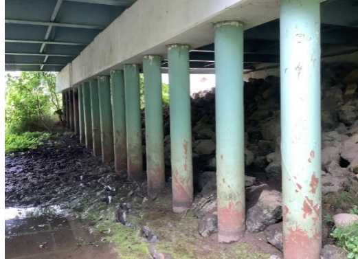
Figure 7-9: Steel spiral-welded piles with a reinforced concrete cap.
