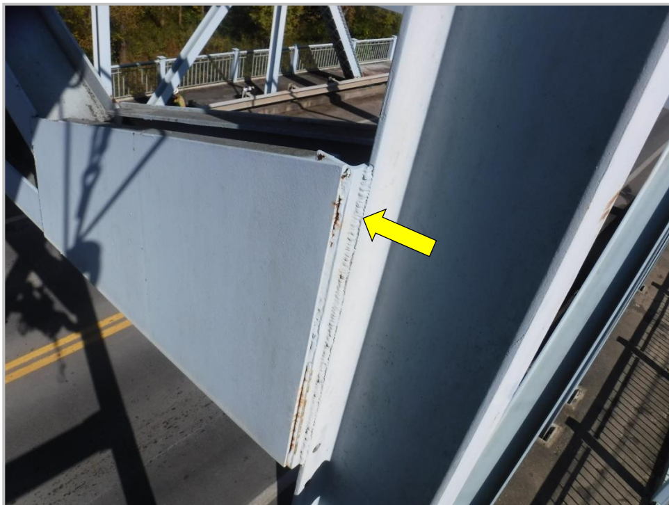
Photo 1 – Sway bracing connection angle attached by fillet welds with no transition radius ( Category E ). U6-L6 of the Right Truss is shown (looking northeast).
