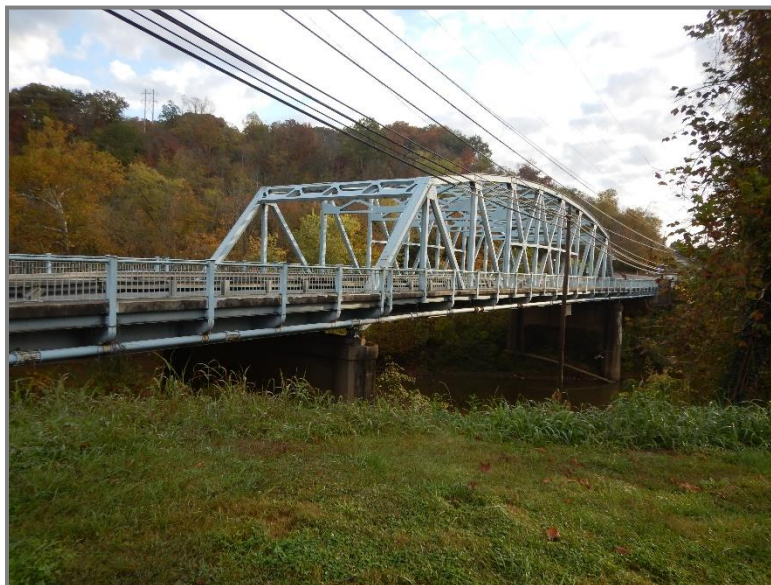
Figure 1 – LAW-7-0240 south elevation looking northeast.
