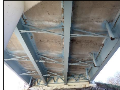
Figure 7-151: Underside of deck in Span 1
