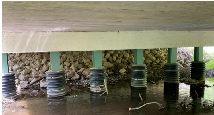
Figure 7-7: H-pile with reinforced concrete cap example.
