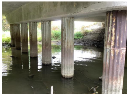
Figure 7-10: Steel fluted pile filled with unreinforced concrete and a reinforced concrete cap.
