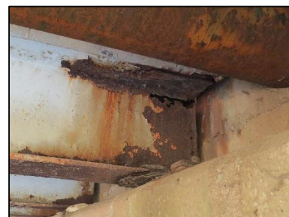
Figure 7-206: Beam 2 at the Rear Abutment
