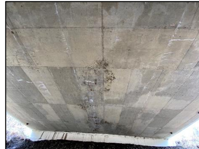
Figure 7-147: Underside of deck in Span
