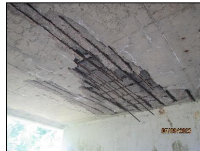
Figure 7-155: Underside of deck in Span 1
