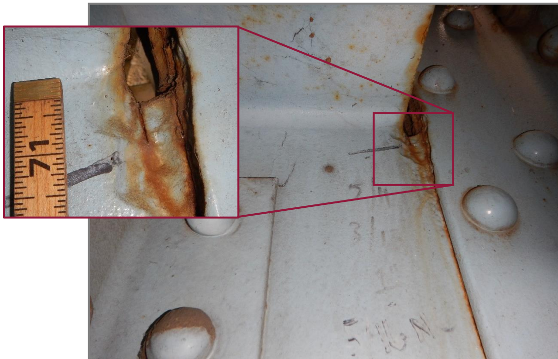
Photo 3 – Overcut in a floorbeam web at the cope at the connection to the truss (looking east at Floorbeam 3 adjacent to the Right Truss).
