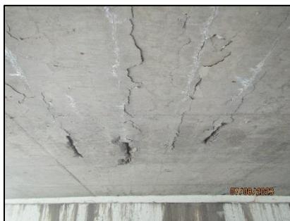
Figure 7-156: Underside of deck in Span 2
