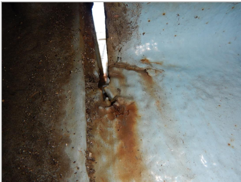
Photo 2 – Cracking in the web of a floorbeam at the upper cope (looking west at Floorbeam 9 adjacent to the Right Truss).
