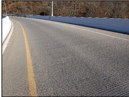
Figure 7-150: Typical wearing surface (Item B.C.01.01 – 6, Satisfactory Condition)
