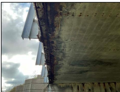
Figure 7-270: Underside of slab along right edge
