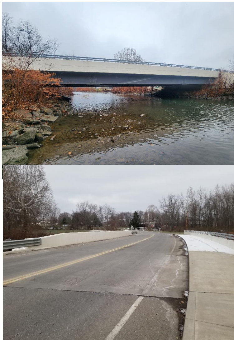
Photo 2 – Approach view to SFN 7661002, looking north.
