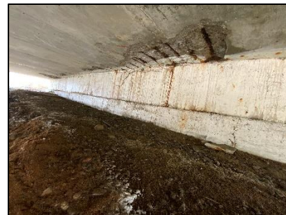
Figure 7-149: Underside of deck in Span
