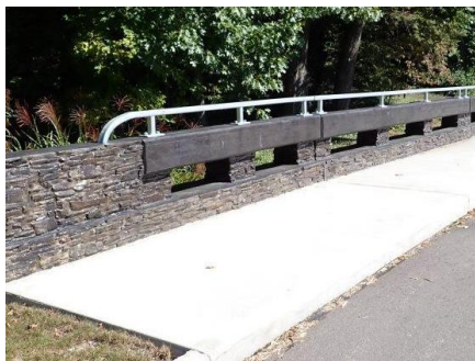
Figure 7-20: Concrete post and rail with metal handrail along top edge.
