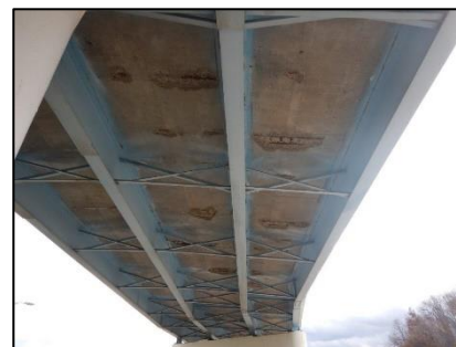
Figure 7-153: Underside of deck in Span 3
