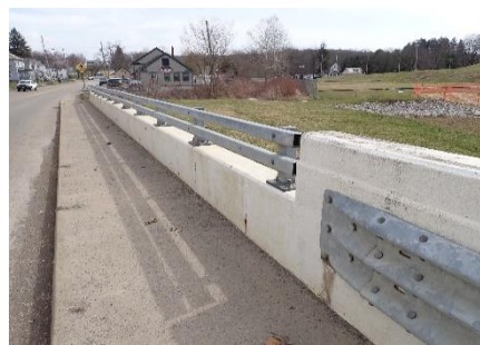
Figure 7-16: Concrete railing with twin steel tube railing.
