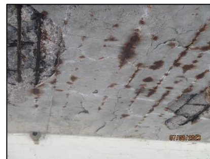
Figure 7-157: Underside of deck in Span 3
