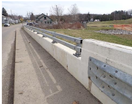
Figure 7-13: Concrete railing with twin steel tube railing.
