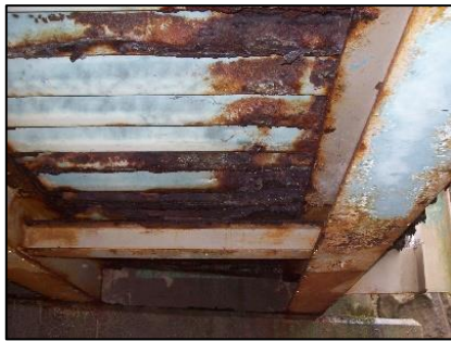
Figure 7-166: Typical underside of deck between beams
