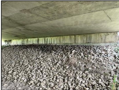
Figure 7-264: Typical underside of slab
