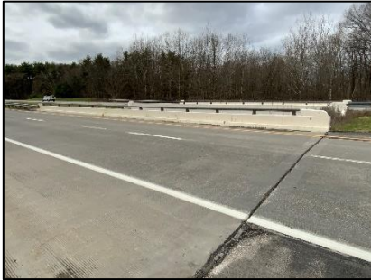
Figure 7-146: Typical wearing surface (Item B.C.01.01 – 7 (Good))
