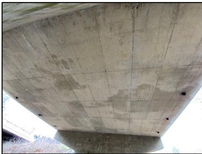
Figure 7-148: Underside of deck in
