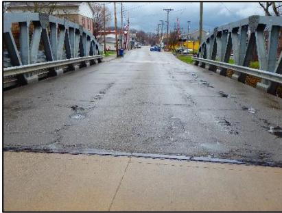
Figure 7-162: Typical wearing surface (Item B.C.01.01 – 5, Fair Condition)
