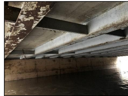
Figure 7-204: Typical underside of framing
