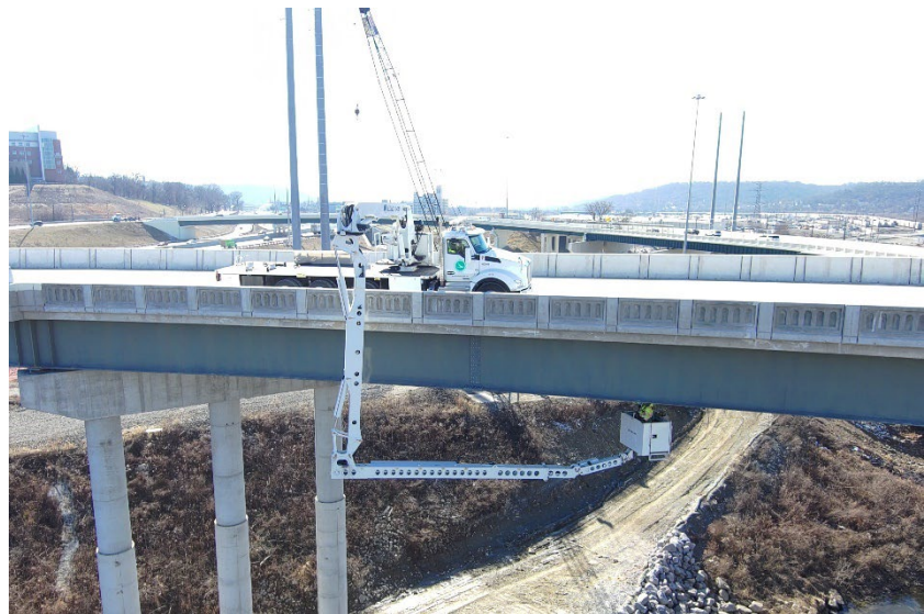
Figure 1 - Snooper Bucket Deployed for Right-Side Operation
