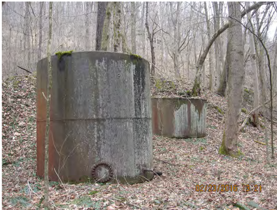
Production tanks for the Farnsworth wells
