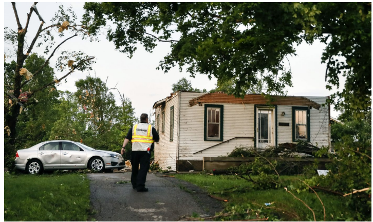
Figure 37: Storm damage litters a residential neighborhood, in Dayton, Ohio, Tuesday, after a rapid-fire line of apparent tornadoes tore across Indiana and Ohio overnight. The storms were packed so closely together that one crossed the path carved by another.
