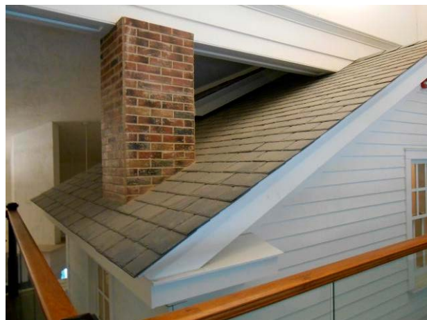
The roof of the Poland Union Seminary is inside the Poland Library and can be seen clearly from the mezzanine.
