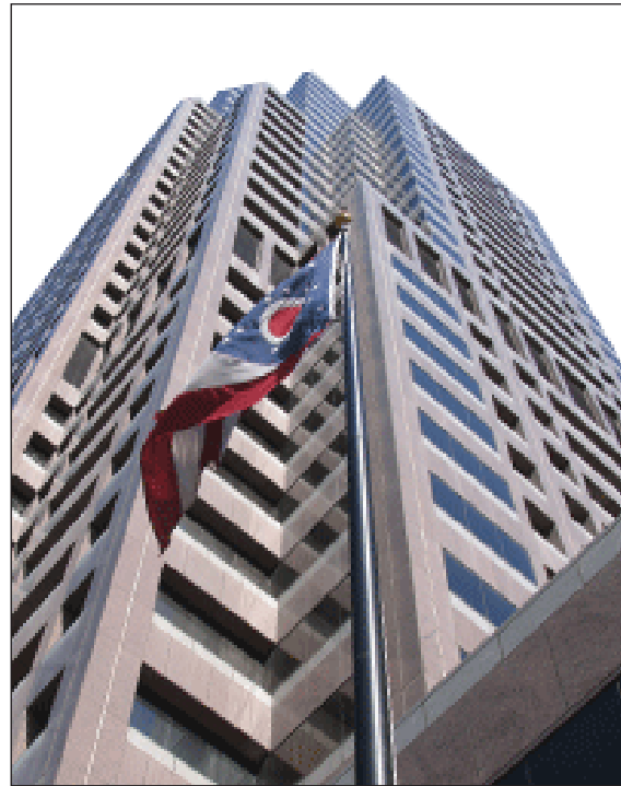
William Green Building Ohio Bureau of Workers' Compensation and Ohio Industrial Commission. Source: https://www.ic.ohio.gov/
