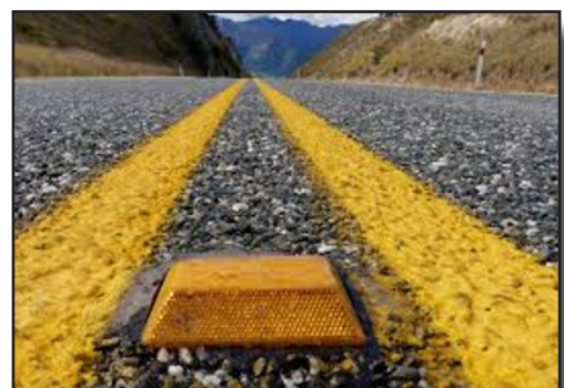
Example of raised pavement marker
