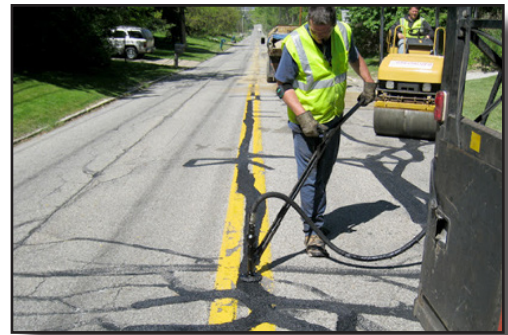
Example of crack sealant project
